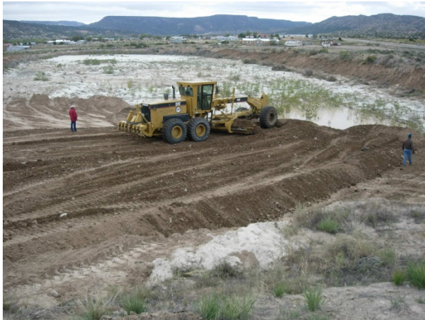
Application of cover soil over the tailings impoundment
