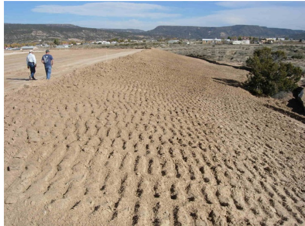
Tailings dam out slope after regrading and covering
