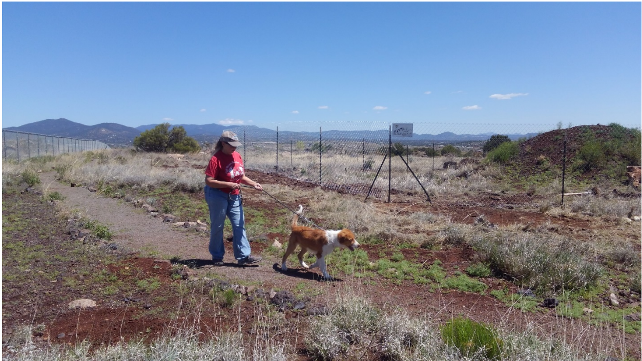
A Humane Society worker safely walks one of the dogs next to newly installed fence.
