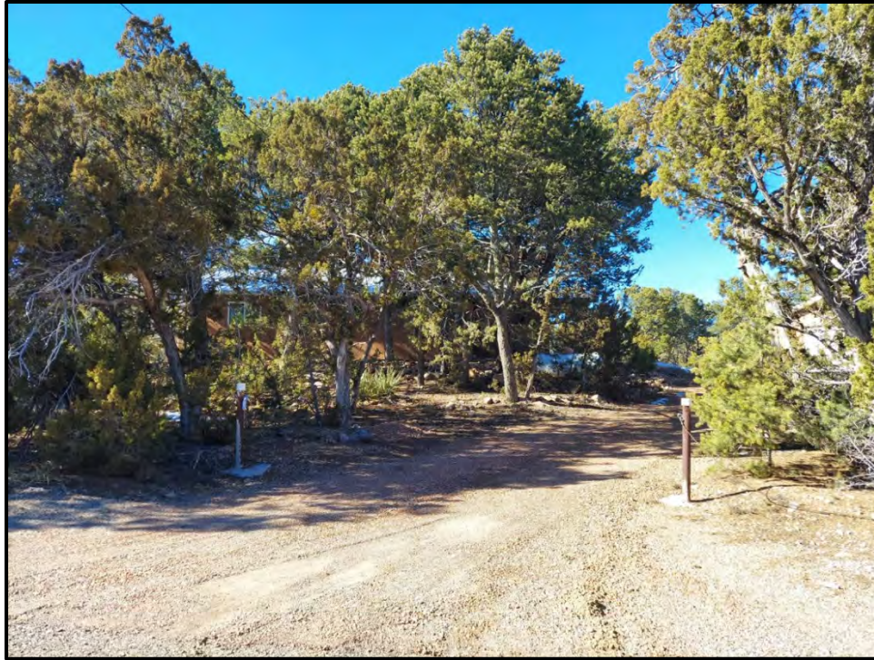
Figure 2.11. Example of an unsurfaced road with overhanging vegetation.
