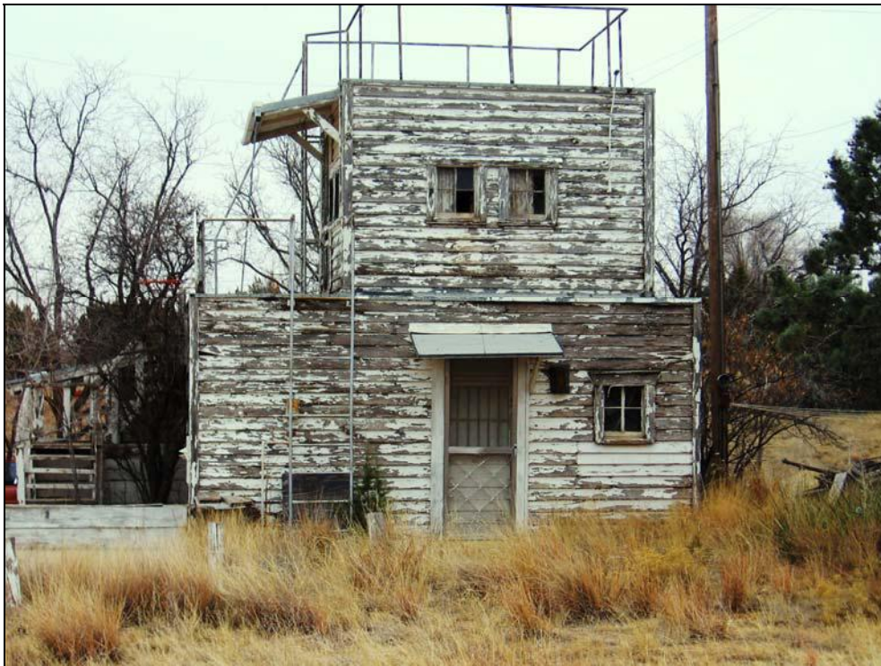
Figure 4.2. Structure with potential extreme combustibility.
