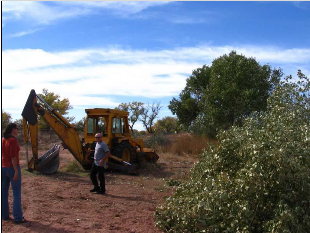
Figure 2.5. Ongoing removal of Russian olive and saltcedar in De Baca County.
