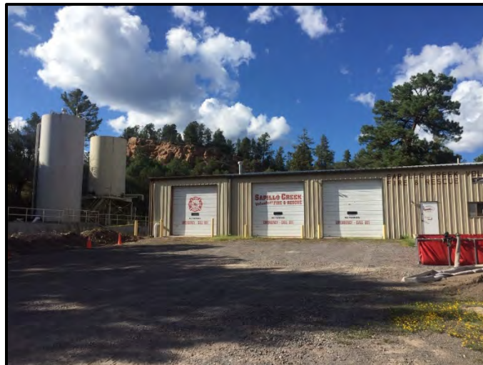
Figure 2.16. Water storage tanks at the Sapillo Creek VFD.
