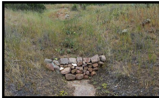
Image 3 a check dam stabilizes soil behind it
