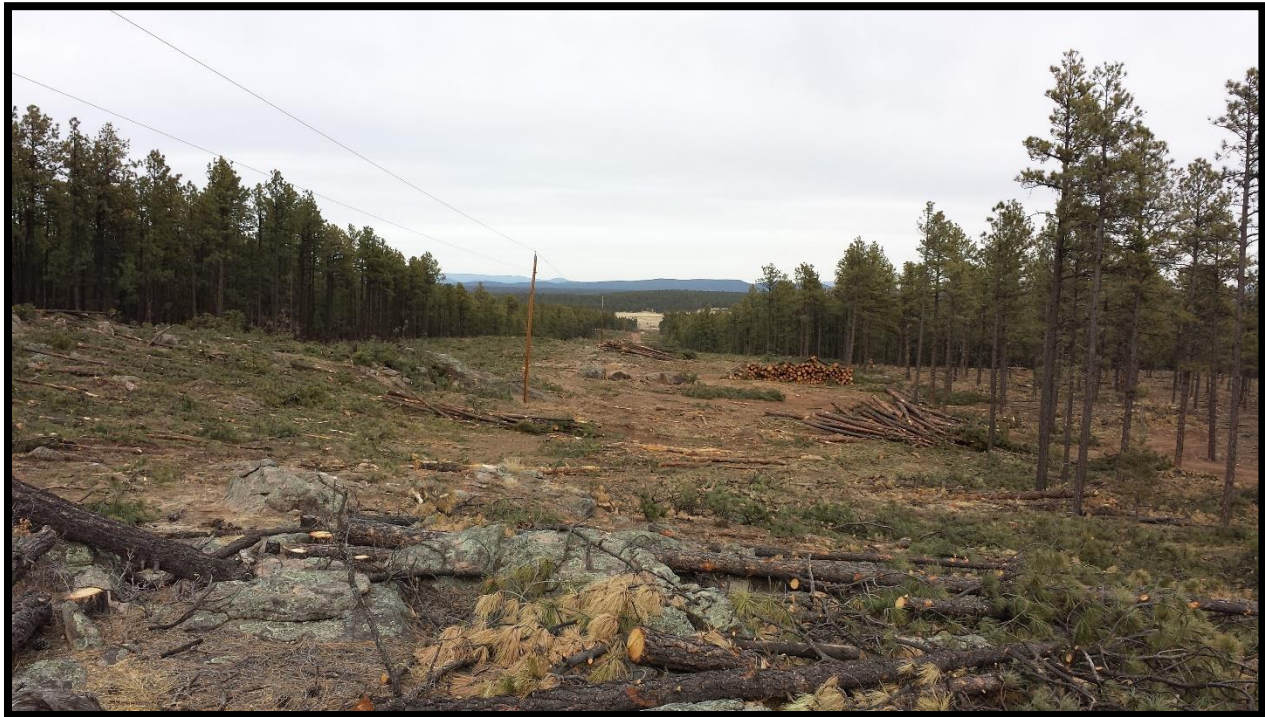
Image 2 - Example of fuels reduction along power line corridor
