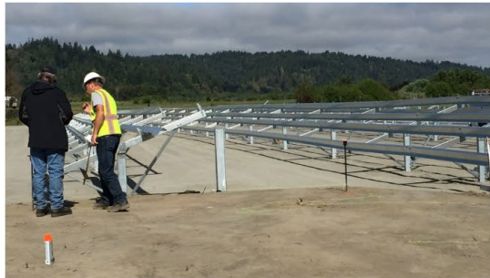
Workers installing the racking for the Blue Lake Rancheria's 500-kilowatt solar system in June 2016. The solar system is a cornerstone of the tribe's low-carbon community microgrid project.
