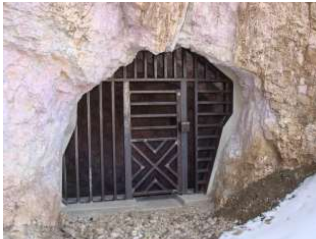
One of the Bat Compatible Closures at the Harding Pegmatite Mine
