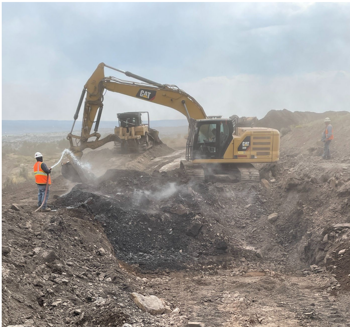
Runyan Construction excavating the burning coal at the Navajo No.1 fire. Water trucks were used to cool the temperature of the piles and suppress excess dust.
