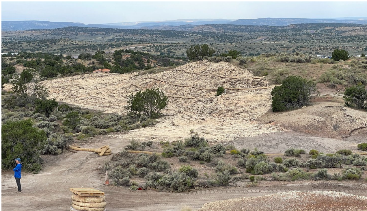
Post-fire mitigation reclamation work at the Navajo No. 1 site. Wood mulch was applied over native seed.
