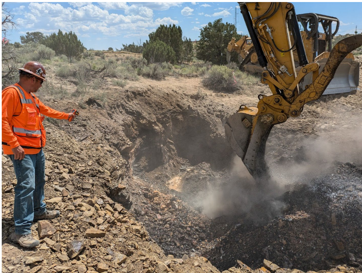
Runyan Construction excavating the burning coal at the Enterprise Brown fire. Temperature measurements were taken regularly to identify fire limits.
