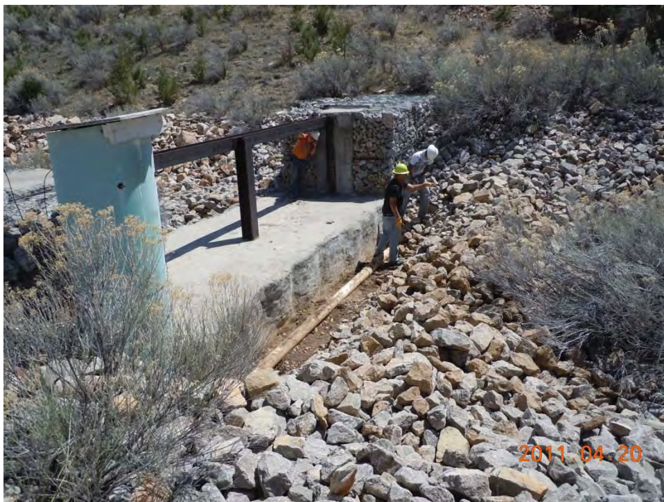
Upgradient face of existing concrete weir with riprap removed.
