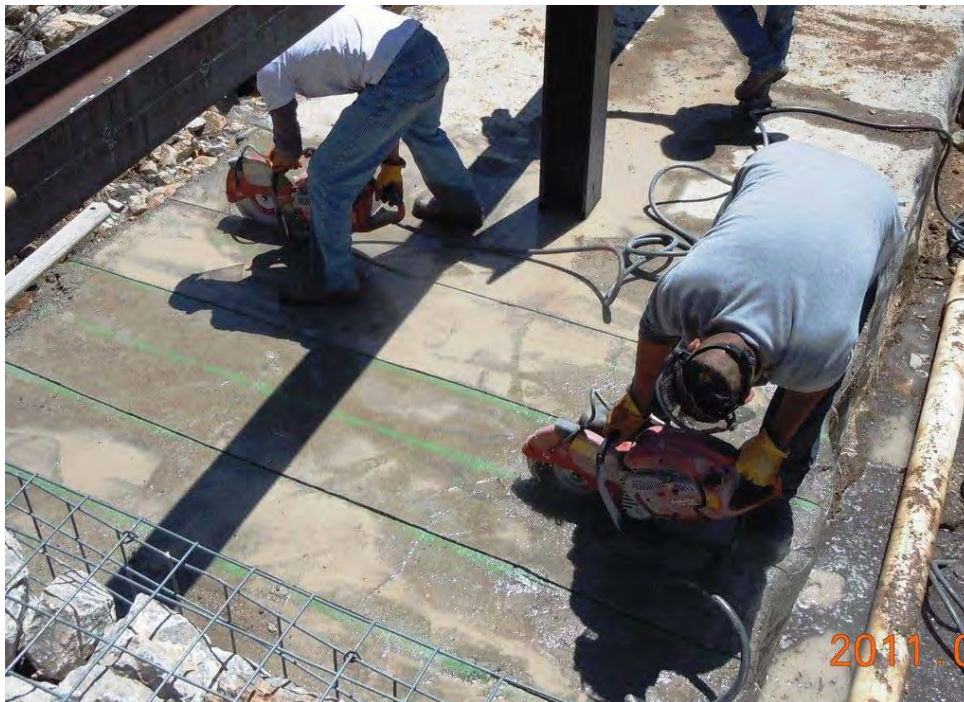
Cutting concrete weir for construction of channel for "V" notch weir
