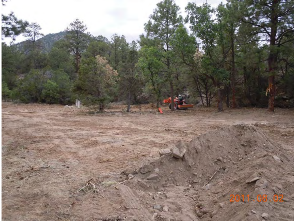
Filling and grading low area upgradient and north of channel.
