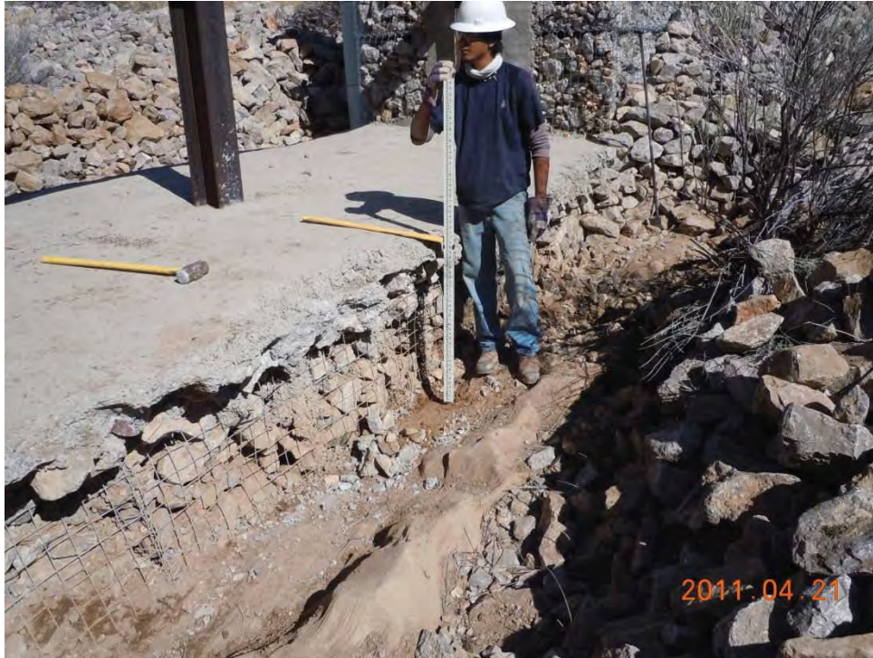
Downgradient side of existing weir. Concrete over gabion basket with riprap.
