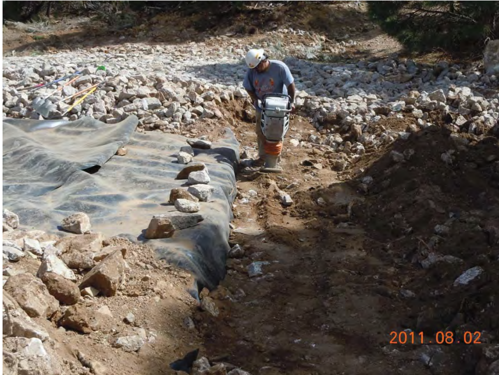
Upgradient liner edge anchor trench near completion with compaction.
