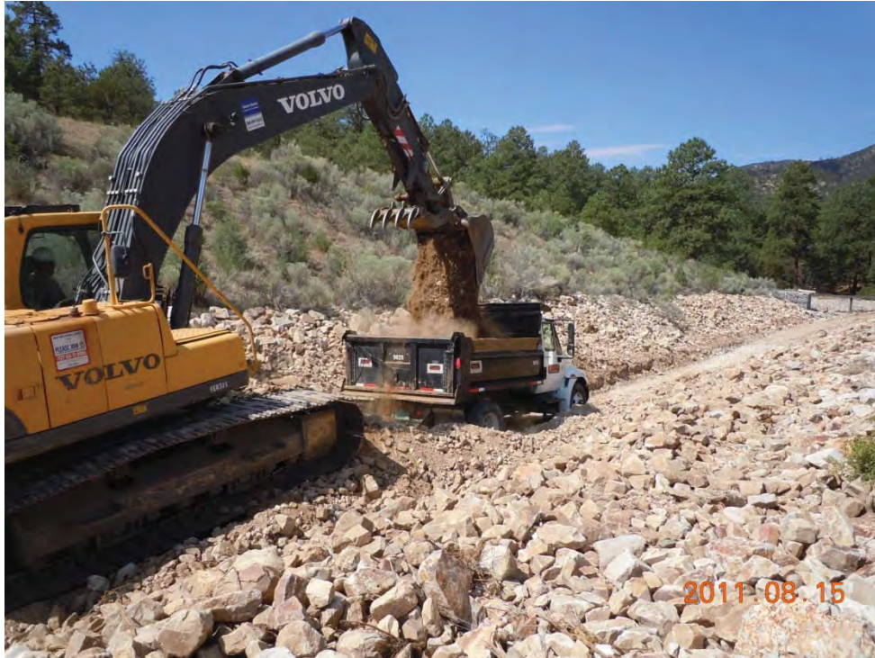
Channel downgradient of weir being excavated to 1% slope.
