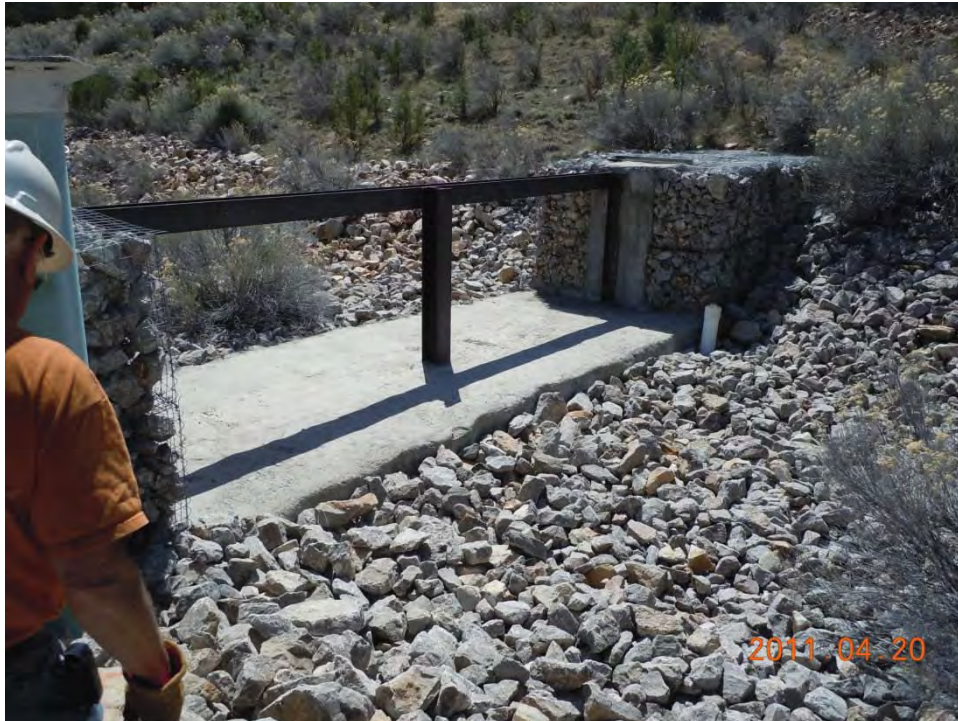
Cunningham Gulch Channel concrete weir with riprap prior to maintenance work.
