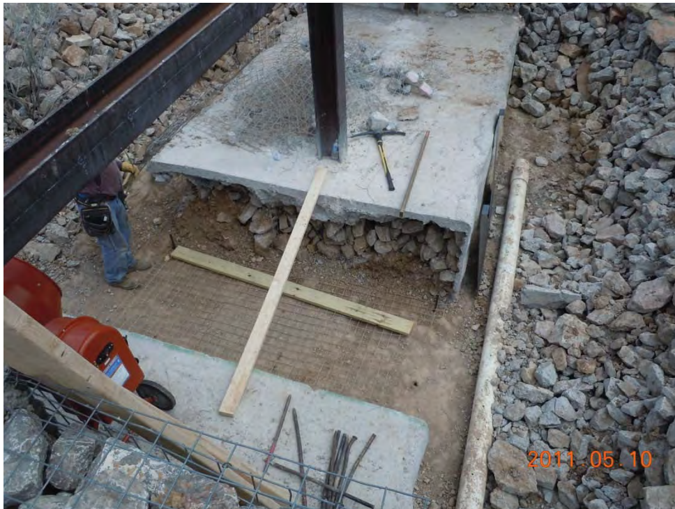
Channel demolition complete and ready for “V” notch weir construction.
