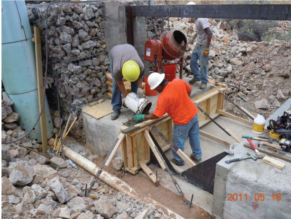
Construction of new “V” notch weir and concrete channel.
