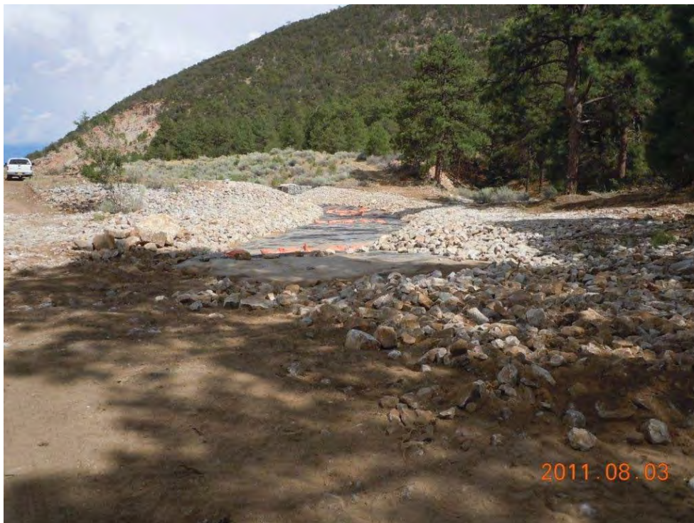
Channel upgradient of weir with HDPE liner installed.
