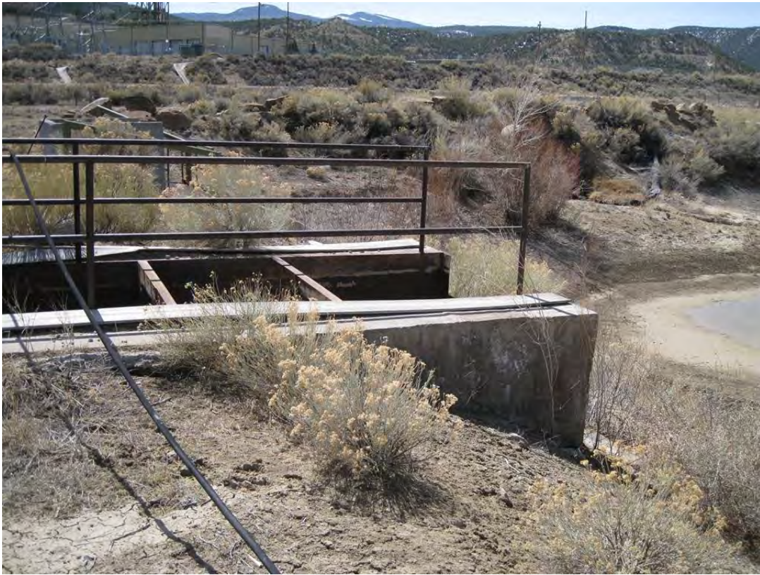
Figure C.2-2 Hydraulic Control Structure on Mine Water Treatment Pond #2 (existing April 2013)
