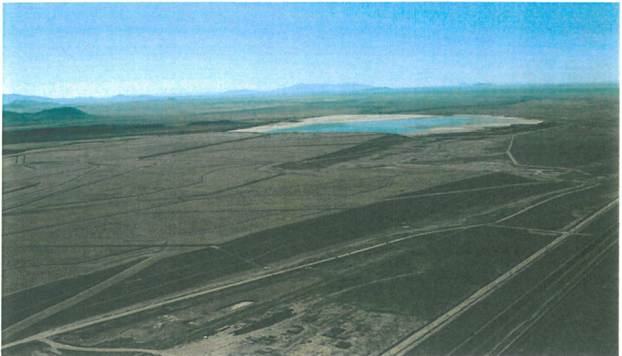
July 27, 2012 - View Northwest to Southeast – Reclaimed areas
