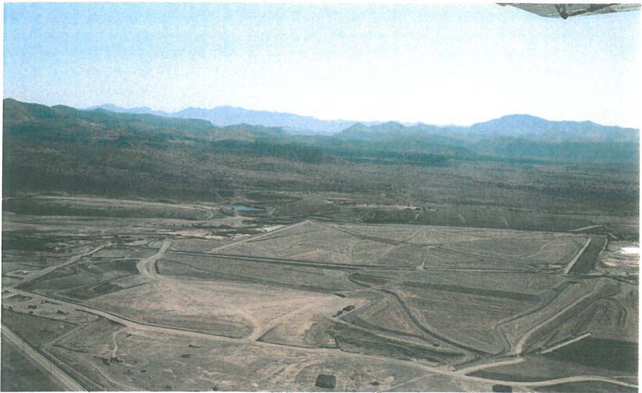
June 6, 2013 - View West to East – of Ponds 1 and 2
