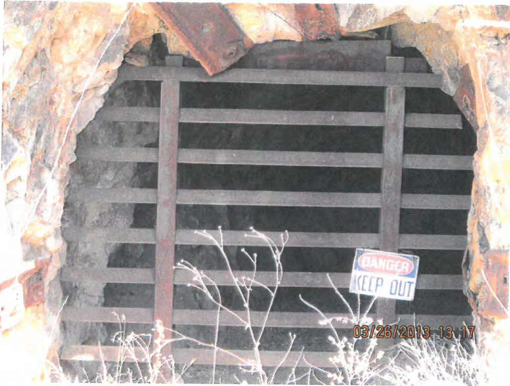
Picture 17: March 26, 2013 – Bat Grate at Virtue Mine
