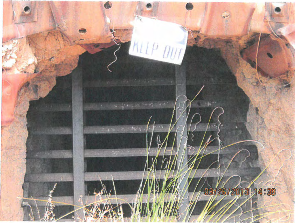
Picture 18: March 26, 2013 – Bat Grate at Jersey Lily Mine
