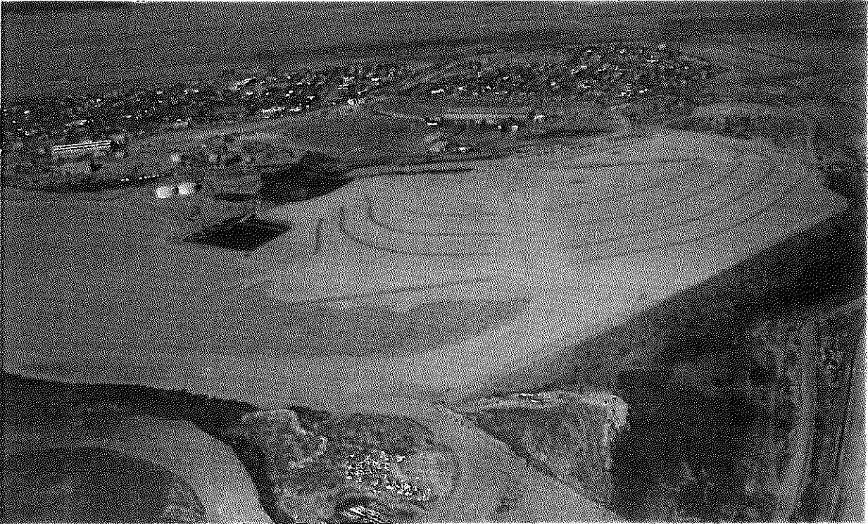
September 10, 2014 – View East to West – Lake One and Slag Pile
