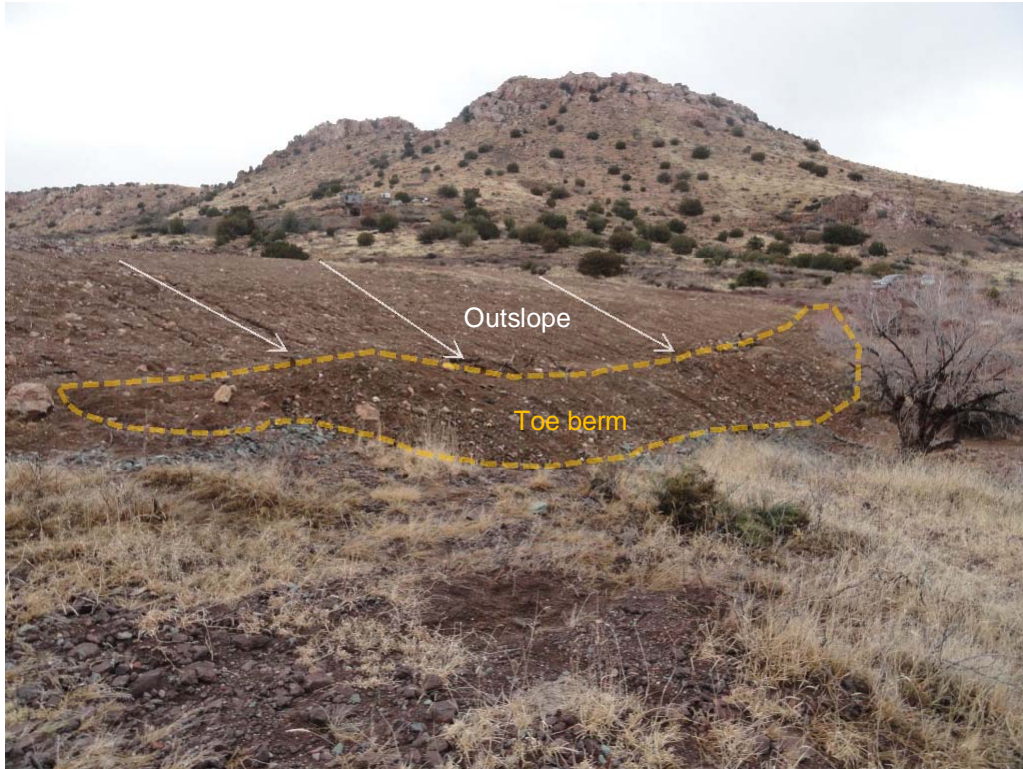
Toe berm at base of outslope of tailings reclamation; looking approximately NE
