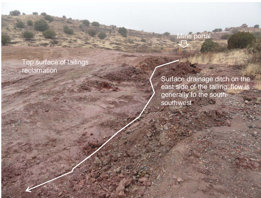
Drainage trench along east side of tailings reclamation; looking approximately North
