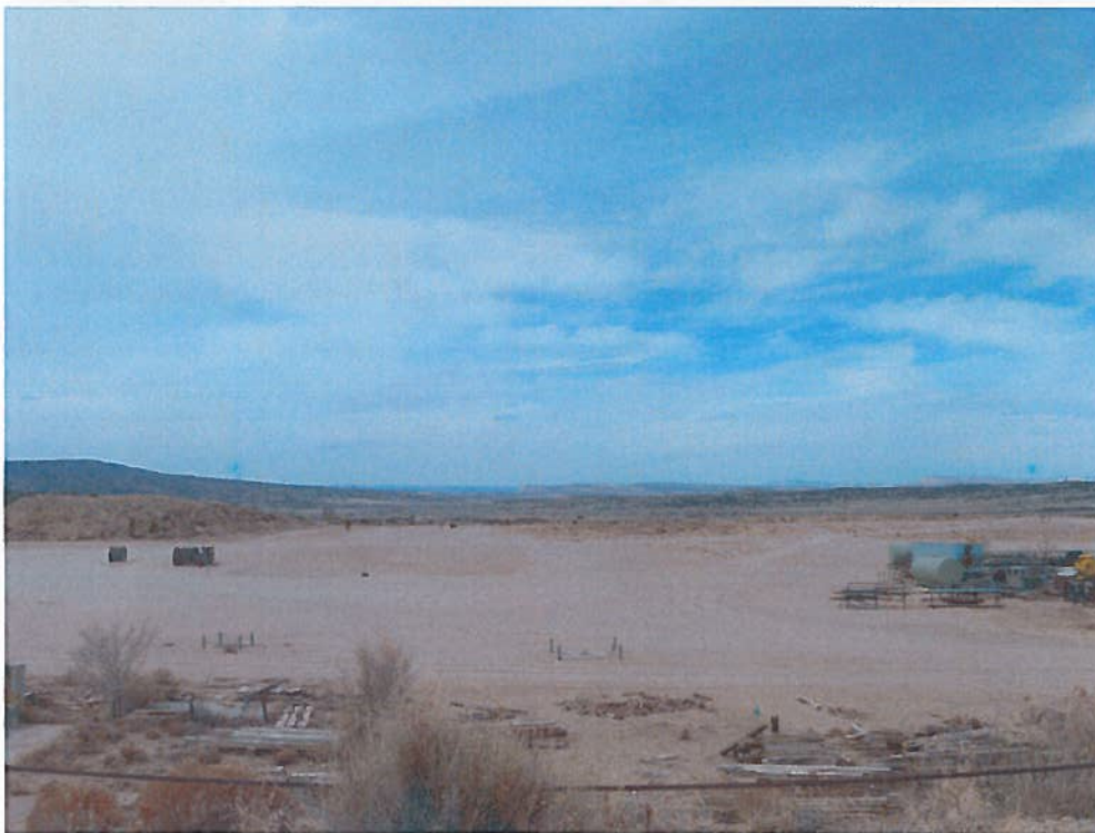
North Top Surface of Waste Rock Pile on April 5, 2018 (looking west)
