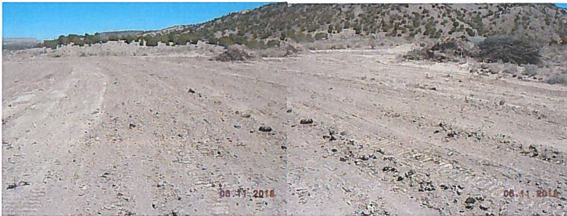
West Portion of Borrow Area grubbed for clay liner source material
