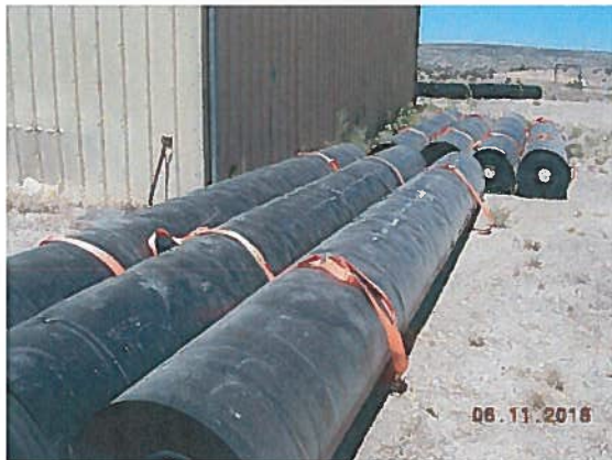
Rolls of HDPE Liner and Geo-mesh staged at Water Treatment System
