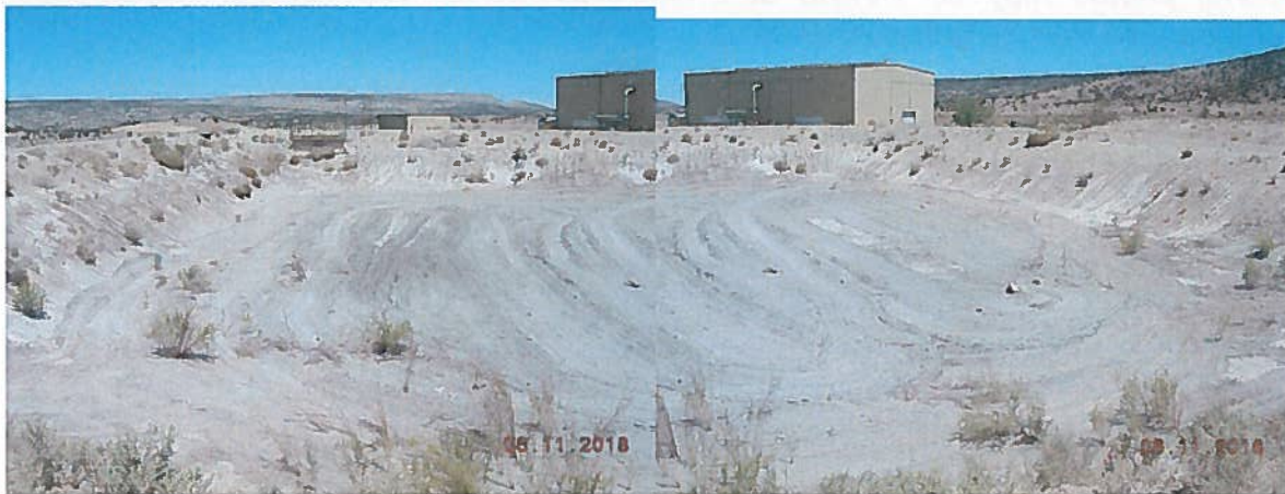
Water Treatment System Pond 2
