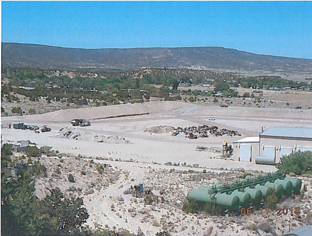
Top Surface of Waste Rock Pile on June 11, 2018 (looking southwest)
