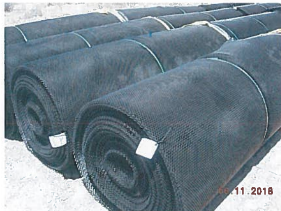
Rolls of HDPE Liner and Geo-mesh staged at Water Treatment System
