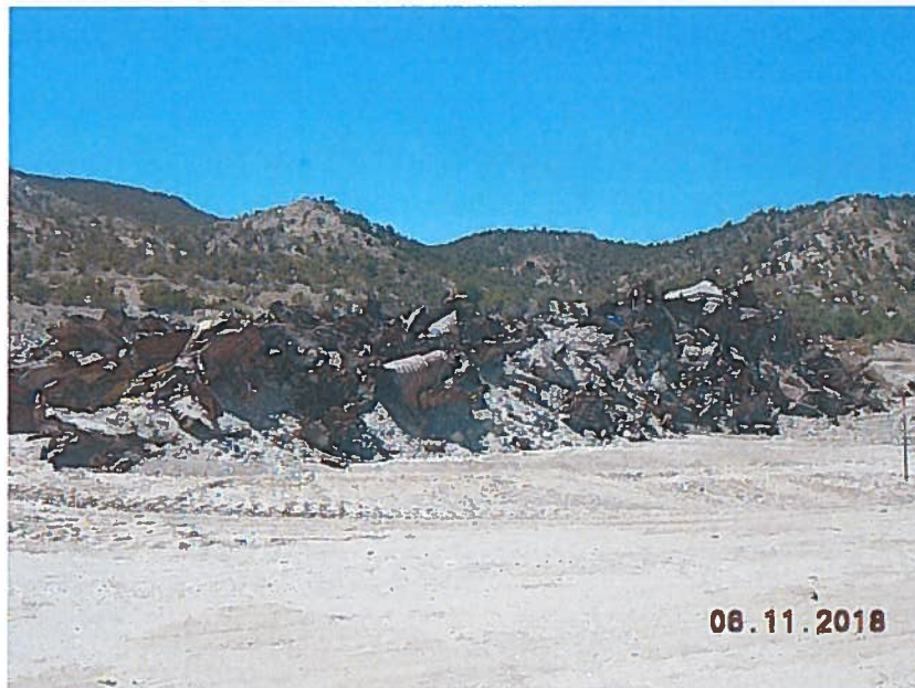
Vent bag and ductwork debris excavated from the Waste Rock Pile
