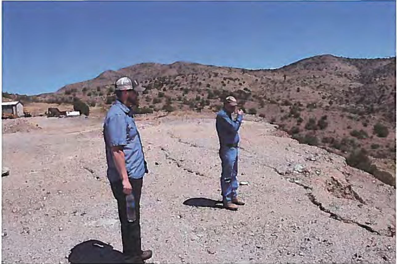
Figure 1: Tension Cracks at the Top of the DMS Failure
