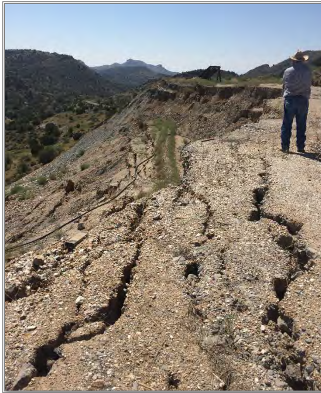
Photograph 3: Surface Tension Cracks
