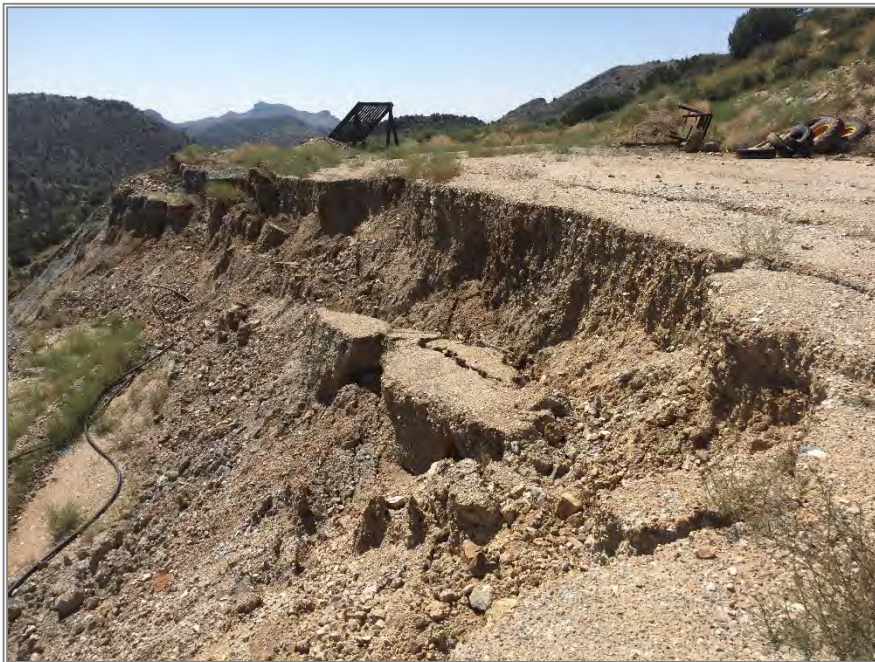
Photograph 2: Highwall and Tension Cracks
