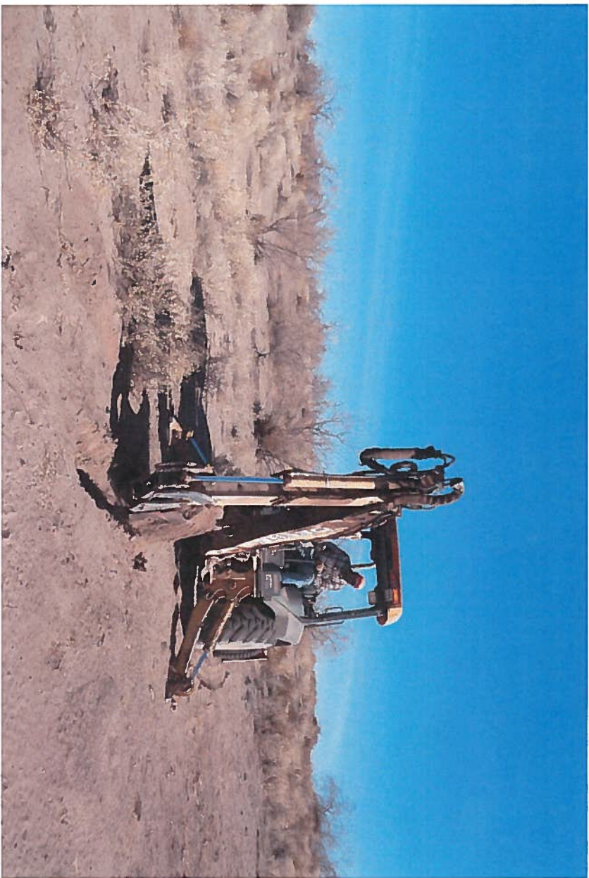
2. Backhoe trench in the northern part of the site. Excavated to 24 inches with no manganese. (February 9, 2018)
