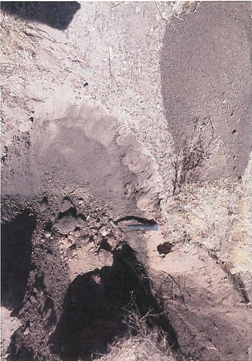
4. Exposed manganese tailing in the northeast berm. (February 9, 2018)
