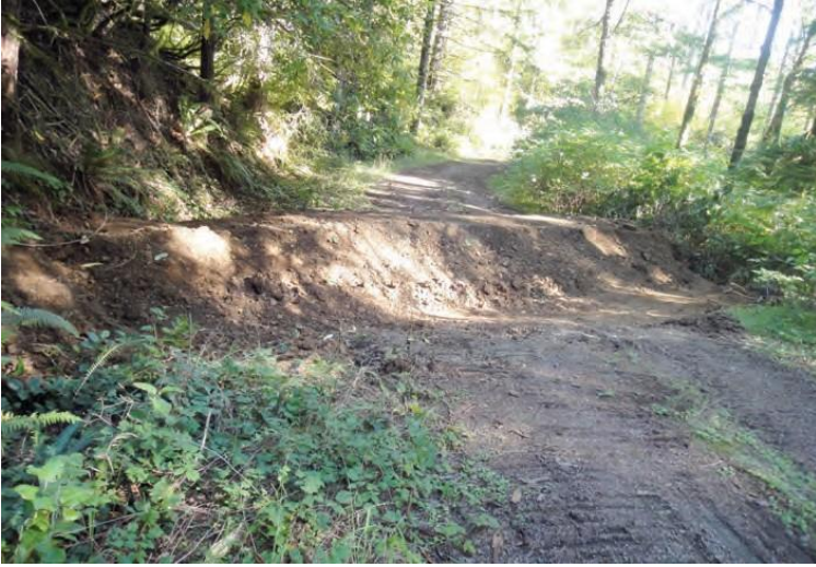
Figure 5 - Typical drivable waterbar.
