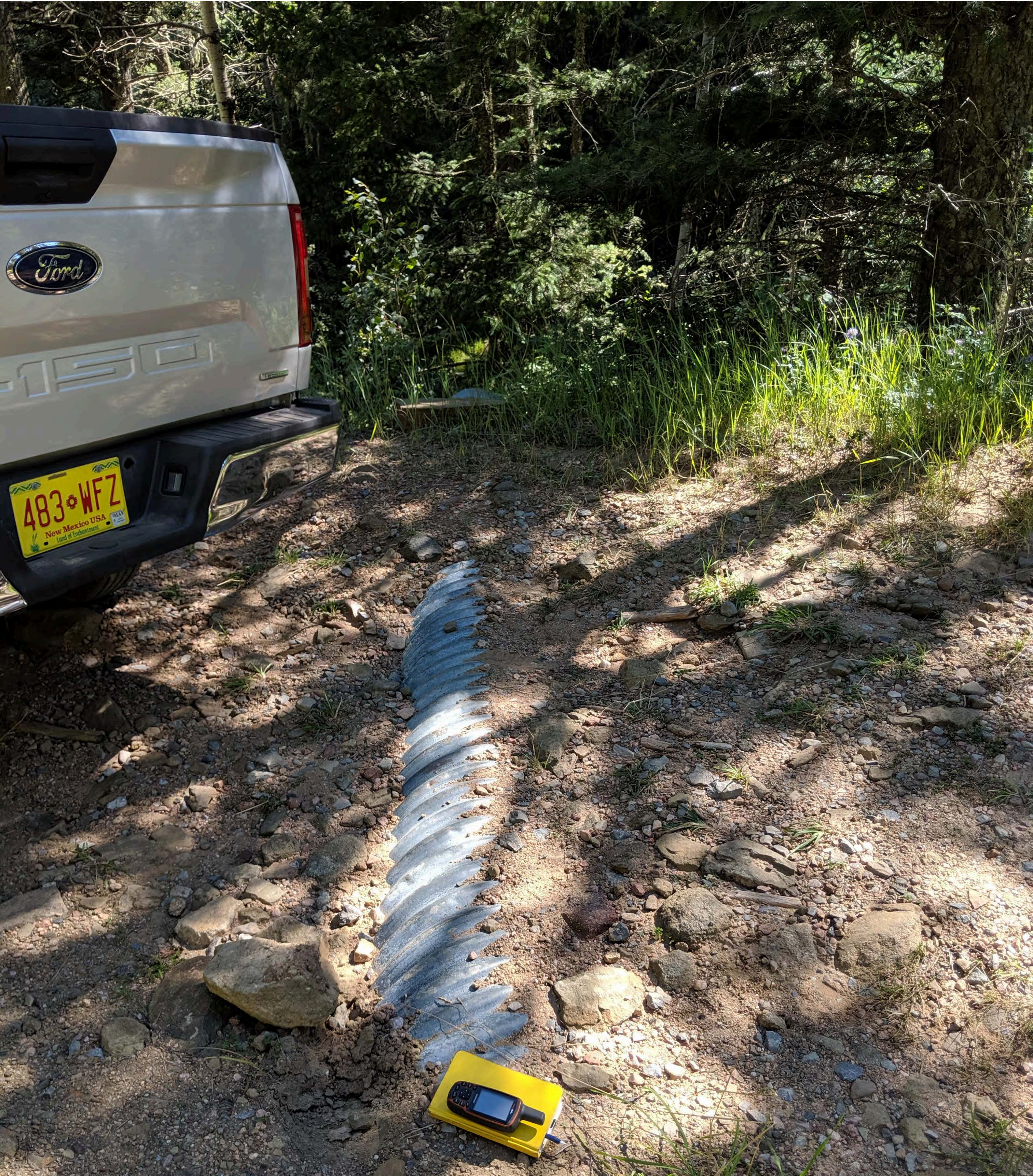
Photo 3: Exposed culvert cross-draining through the roadbed from the out of view cutslope ditch to the fillslope in the distance roadbed.
