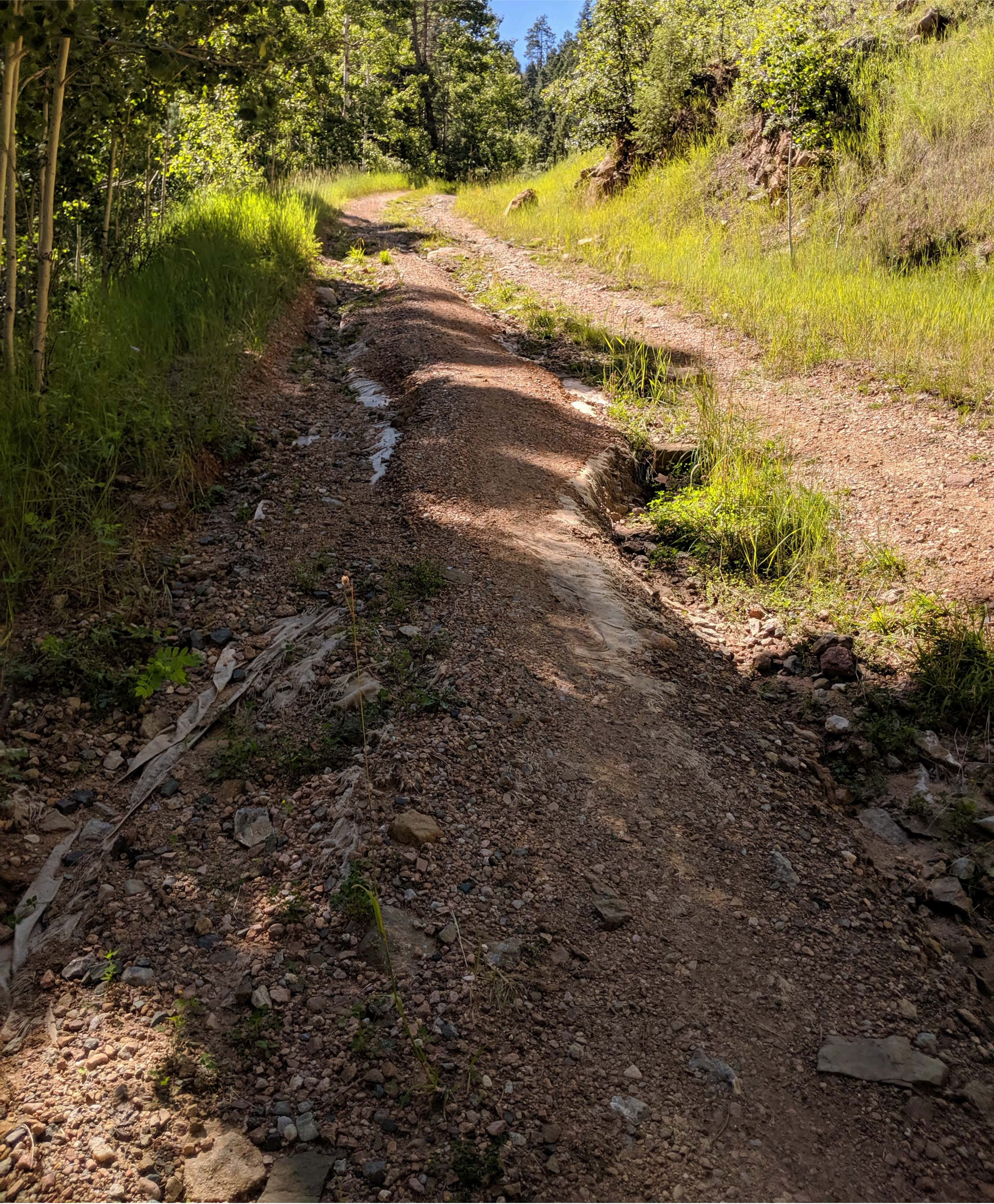
Photo 2: General condition of proposed maintenance segment between FR 192/120 junction and old camp. Roadbed width average of ~5 m, cutslope and fillslope shoulders host healthy vegetation. Ruts and rills, caused by plugged culvert, expose old geotextile beneath aggregate lift.
