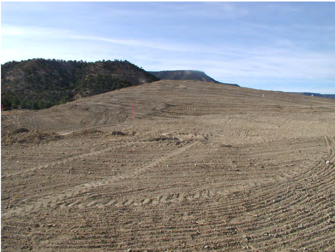
Photo 4 - Final grading of contaminated sediments and soil in disposal cell prior to cover placement
