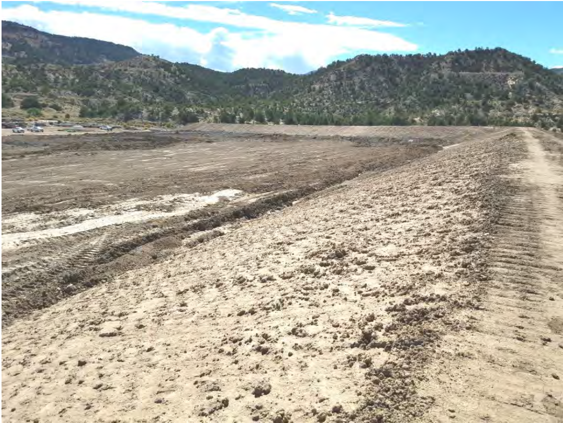
Photo 1 - Clay liner of disposal cell, under construction, from west berm of cell
