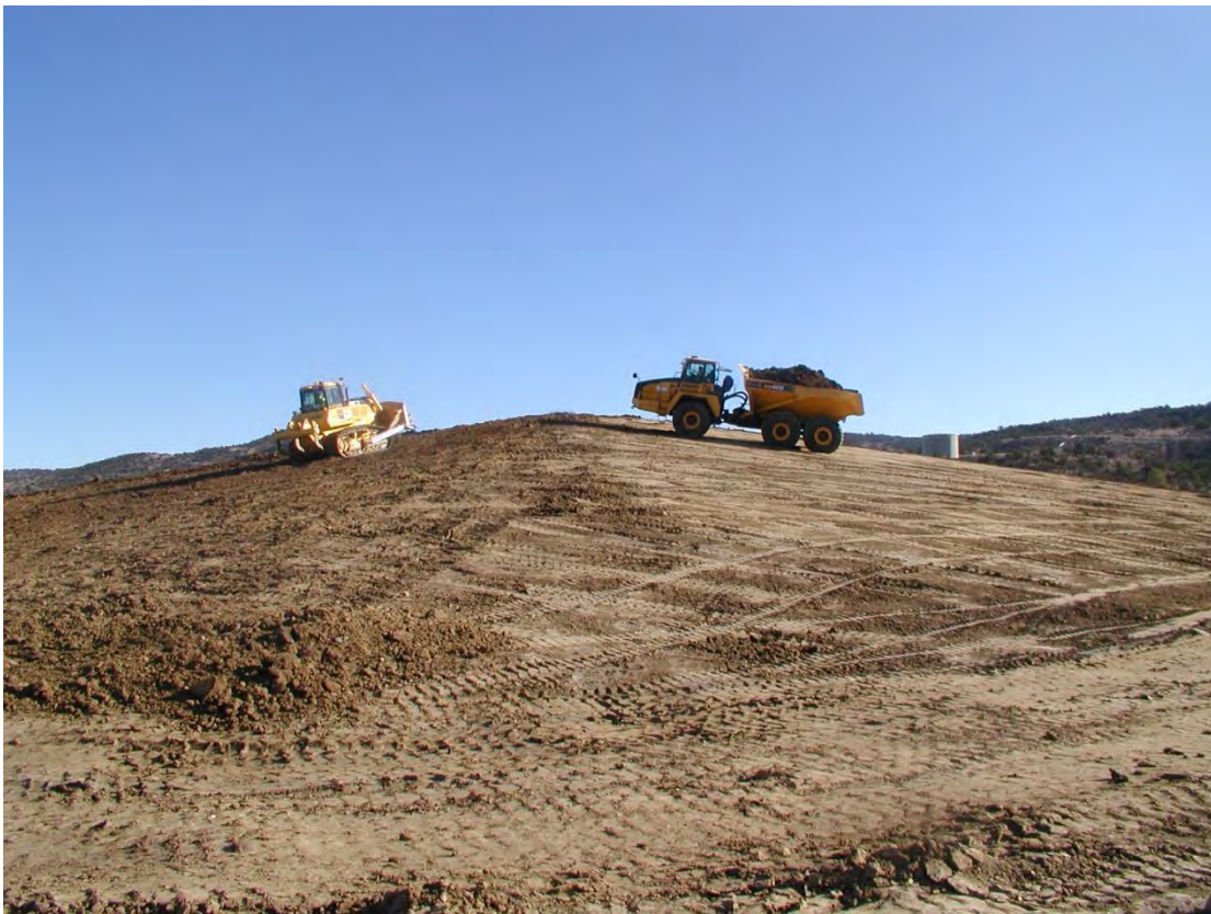
Photo 6 – Cover placement on the top of the disposal cell
