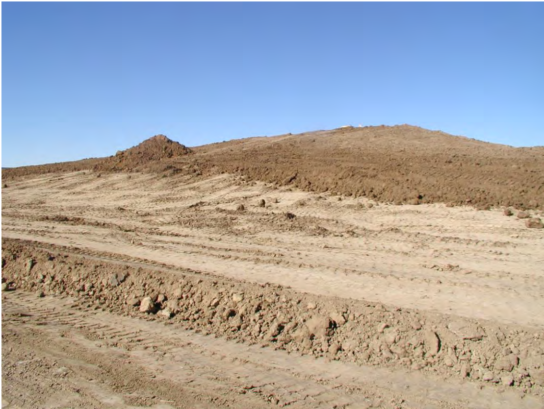
Photo 11 – Growth media being placed on west slope of disposal cell.
