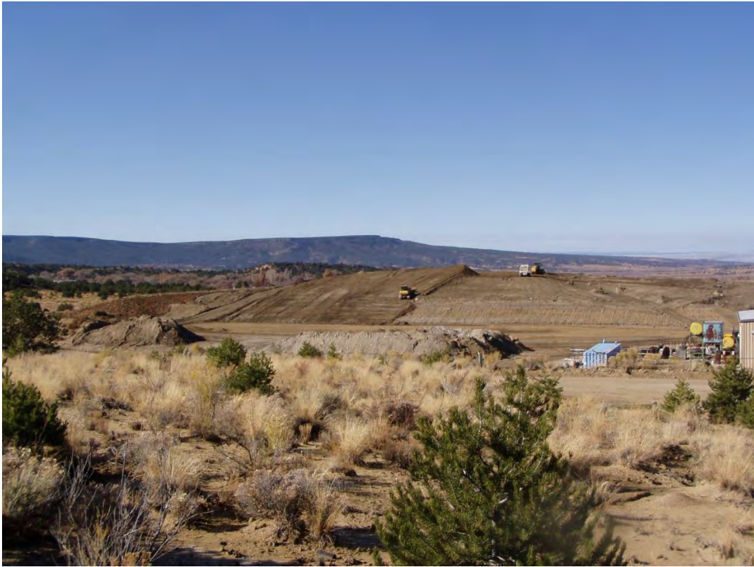
Photo 5 – Radon barrier being placed of the east slope of the disposal cell
