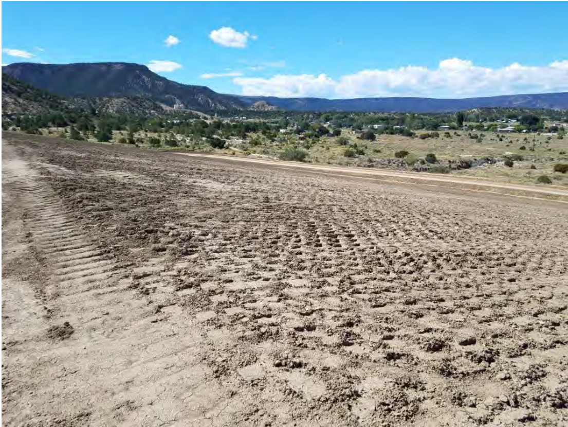
Photo 9 - West slope of waste pile with radon barrier in place
