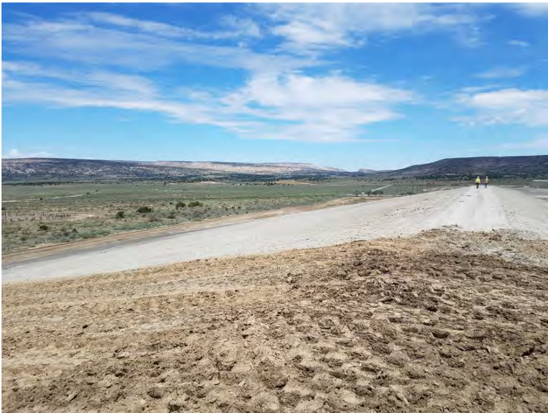
Photo 8 - West slope of waste pile with radon barrier partially in place.
