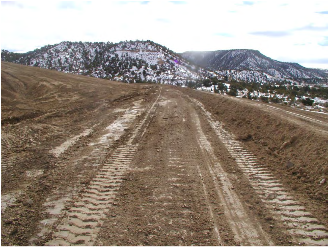
Photo 7 – West slope bench under construction.
