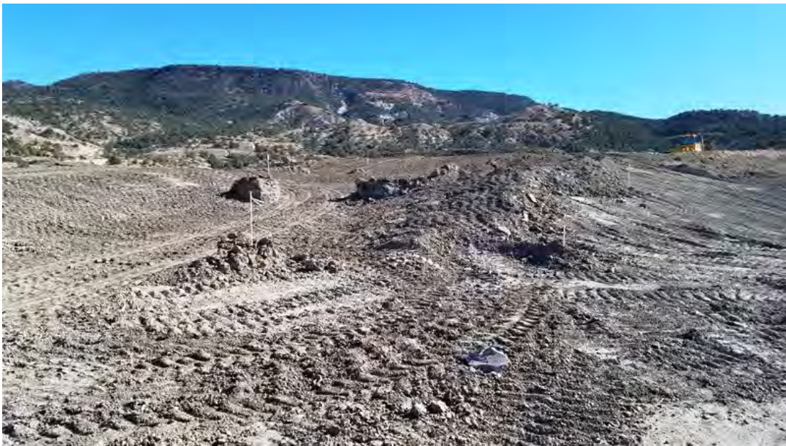
Photo 2 - Contaminated sediment in place in disposal cell, nearing capacity in the 11.5 acre footprint
