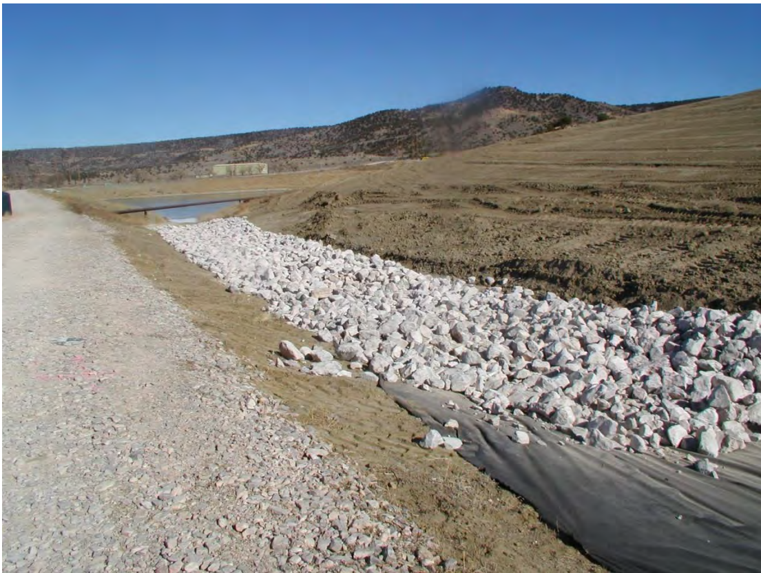
Photo 10 - Riprap placement in drainage ditch at toe of west slope of waste pile
