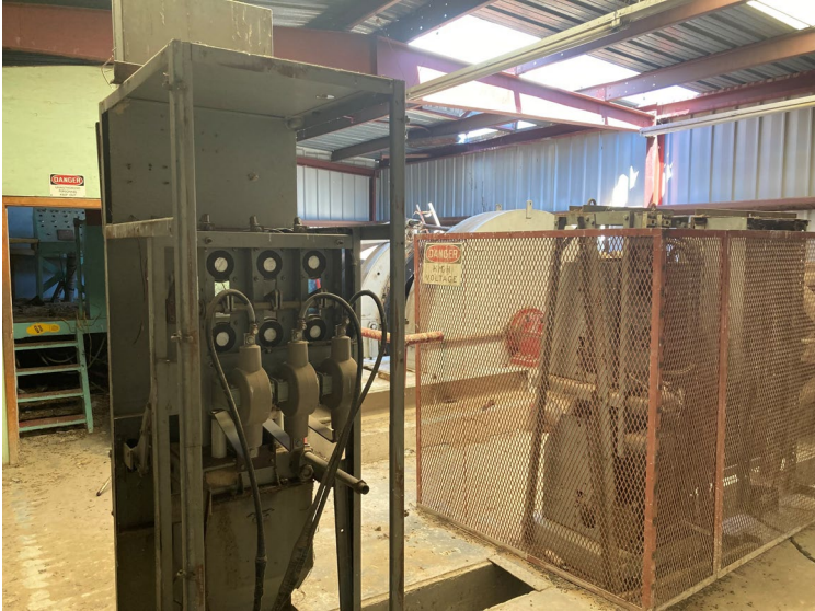
Room 1 (Looking North)
