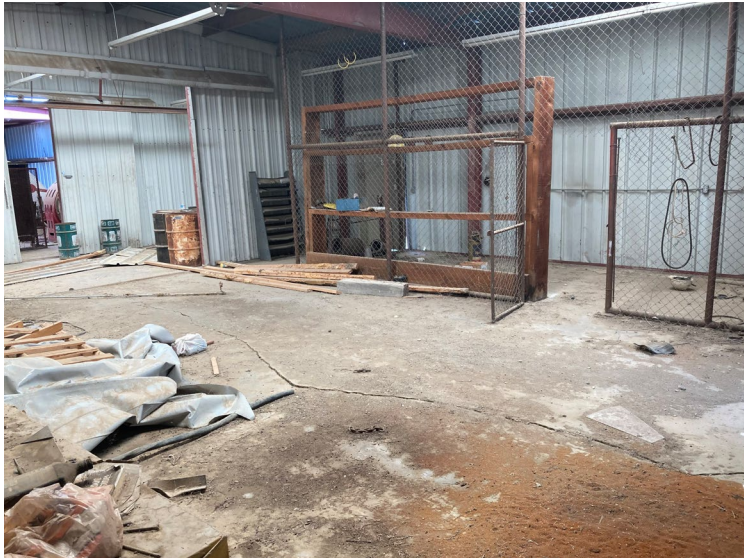
Room 3 (Looking North)
