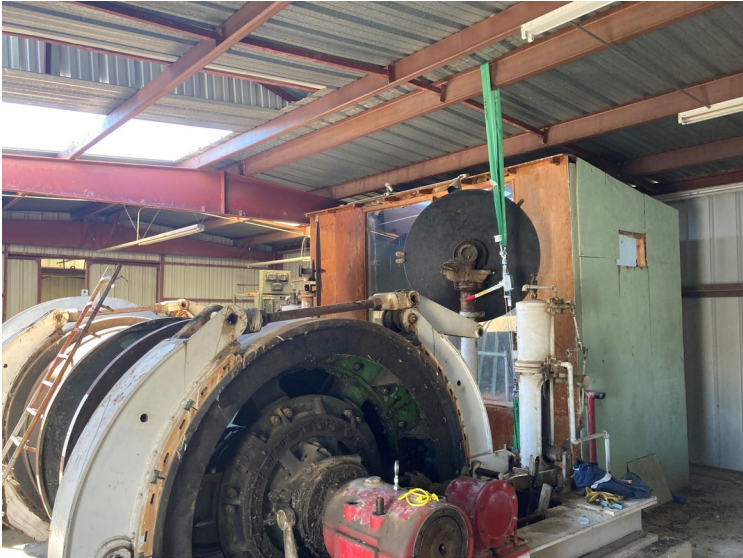
Room 1 (Looking South)
