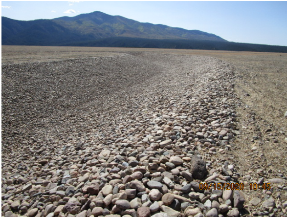
Diversion channel (left) and top surface tailing reclamation (right) at the Questa Mine tailings facility
