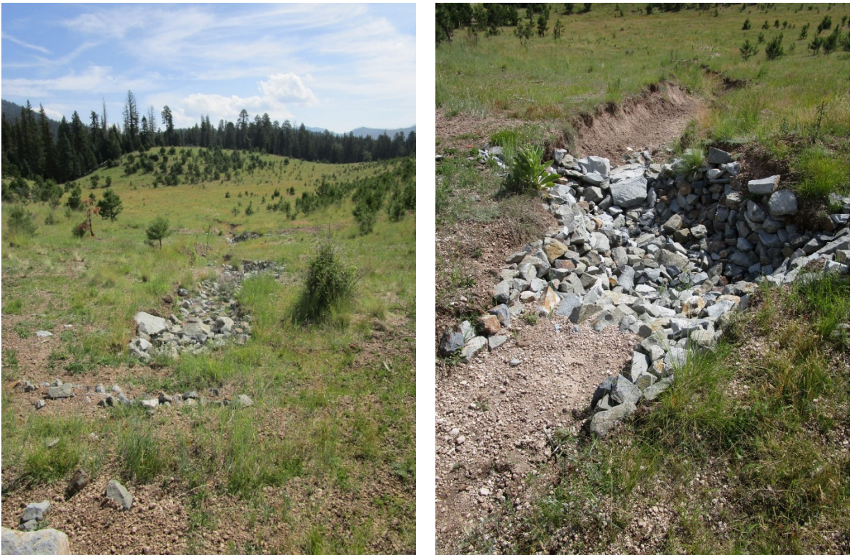
Erosion channel lined with riprap (left) and Zuni bowl created with riprap (right)
