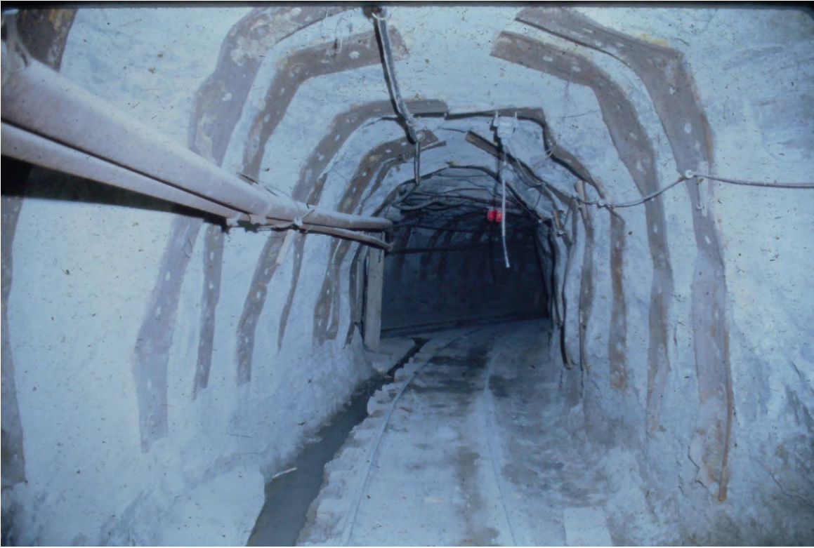
Photo 2-1 Typical mine with dewatering ditch to the left side of the photograph.
