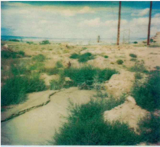
c) End of Sec. 35 sandfill slimes pipeline discharging toward slimes pond 750 feet downhill
