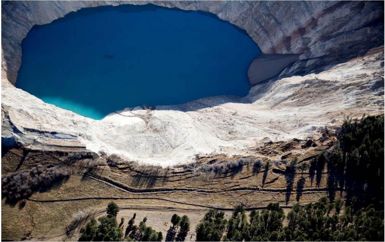
Figure 2. Montana Tunnels Pit Lake and Pit Highwall Unravelling. (Photo by Christopher Boyer)
