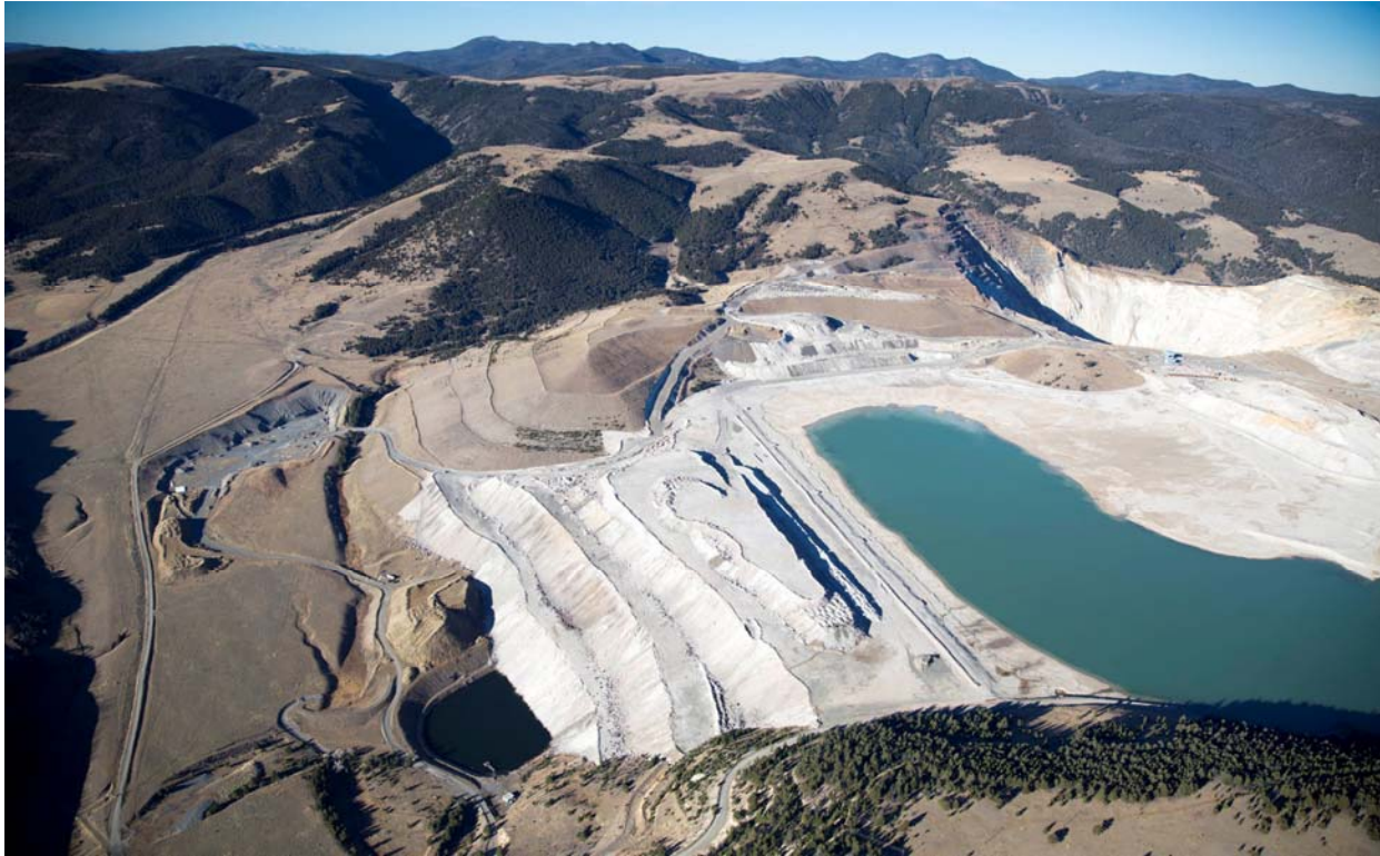
Figure 7. Montana Tunnels Tailings Storage Facility with Waste Rock Pile and Open Pit. (Photo by Christopher Boyer)
