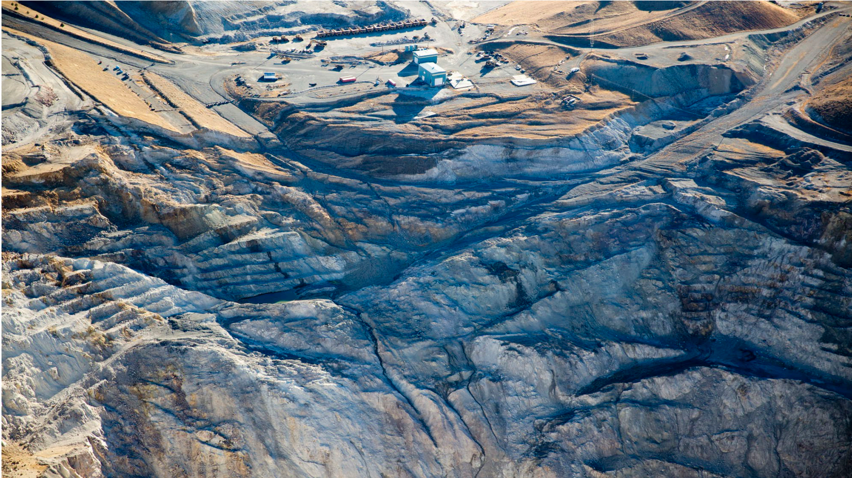
Montana Tunnels Pit Highwall Unravelling. (Photo by Christopher Boyer)
