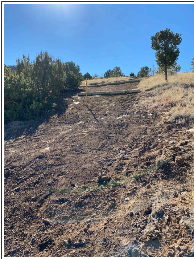
14. WRP location 7 after completion of repairs
