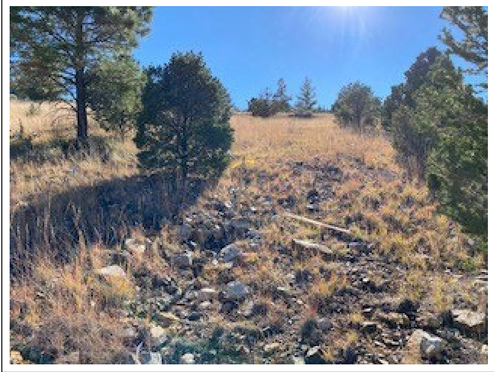
17. WRP location 9 prior to completion of repairs
