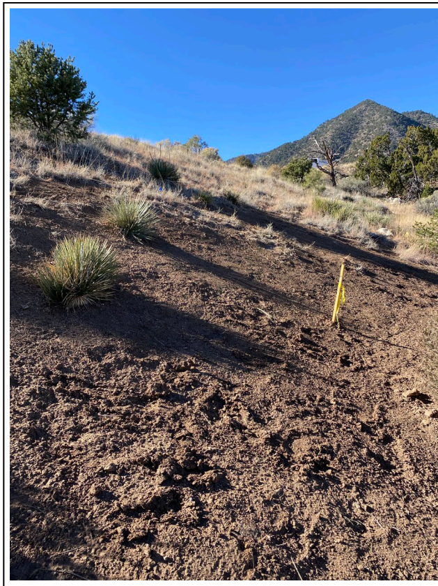
2. WRP location 1 after completion of repairs
