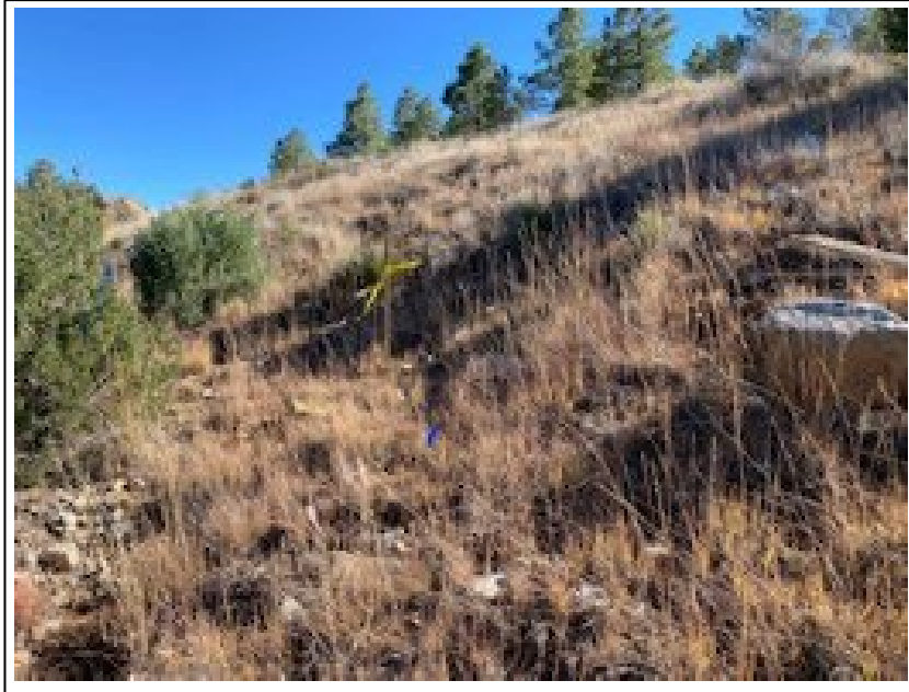
1. WRP location 1 prior to completion of repairs
