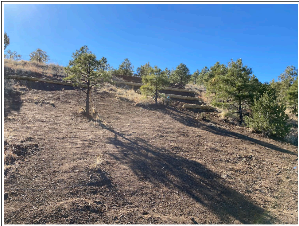
8. WRP location 4 after completion of repairs
