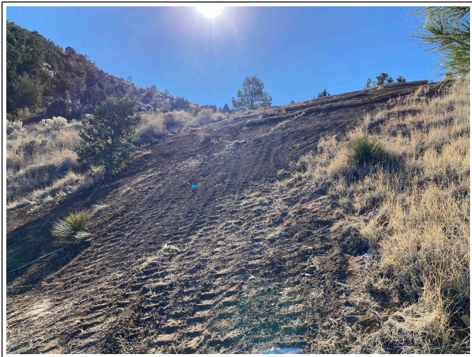
20. WRP location 10 after completion of repairs
