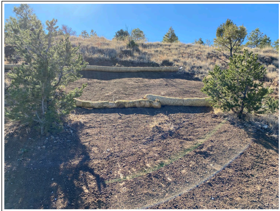
10. WRP location 5 after completion of repairs
