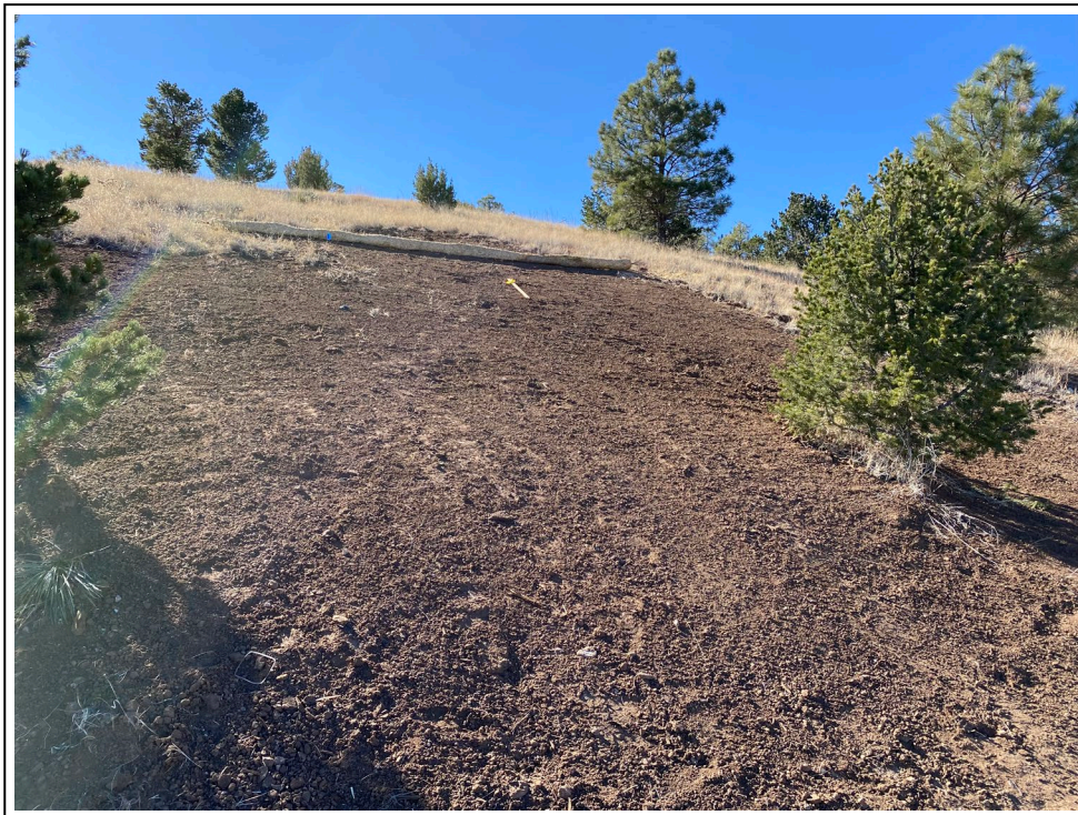
24. WRP location 13 after completion of repairs
