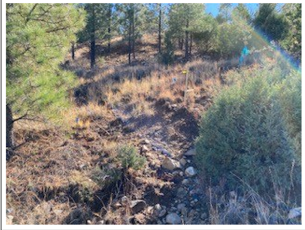
3. WRP location 2 prior to completion of repairs
