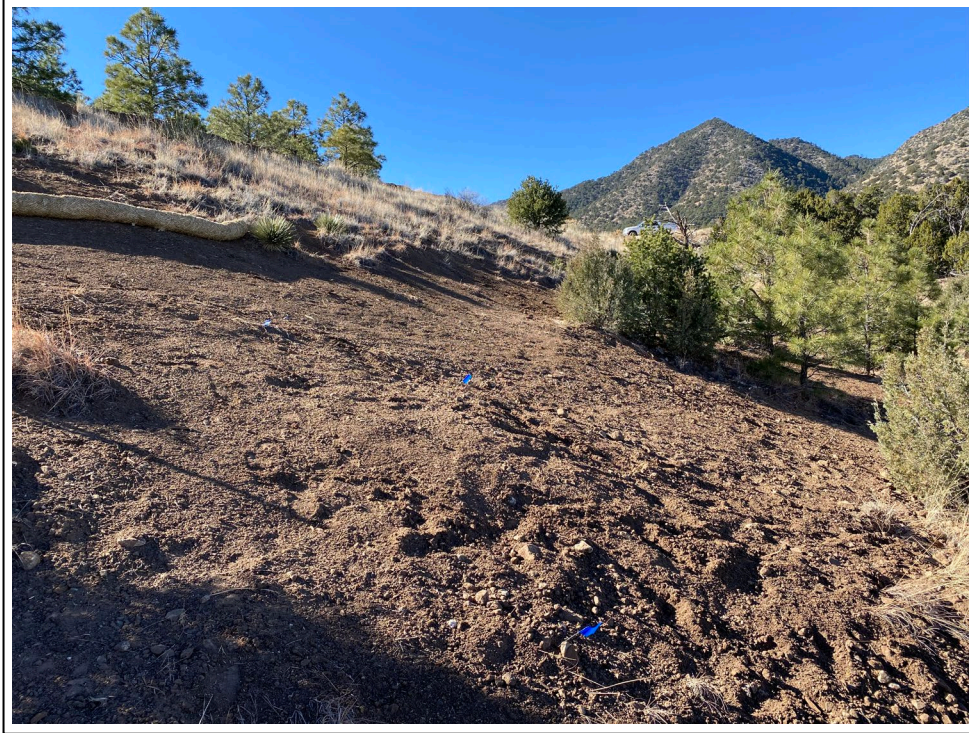
23. WRP location 12 after completion of repairs
