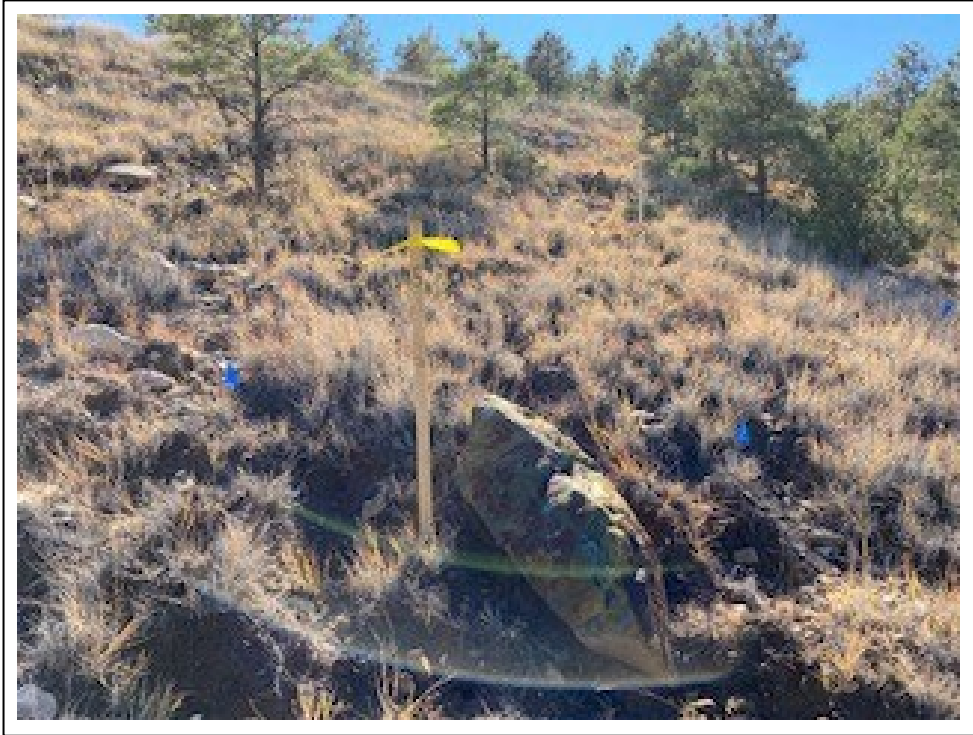
9. WRP location 5 prior to completion of repairs
