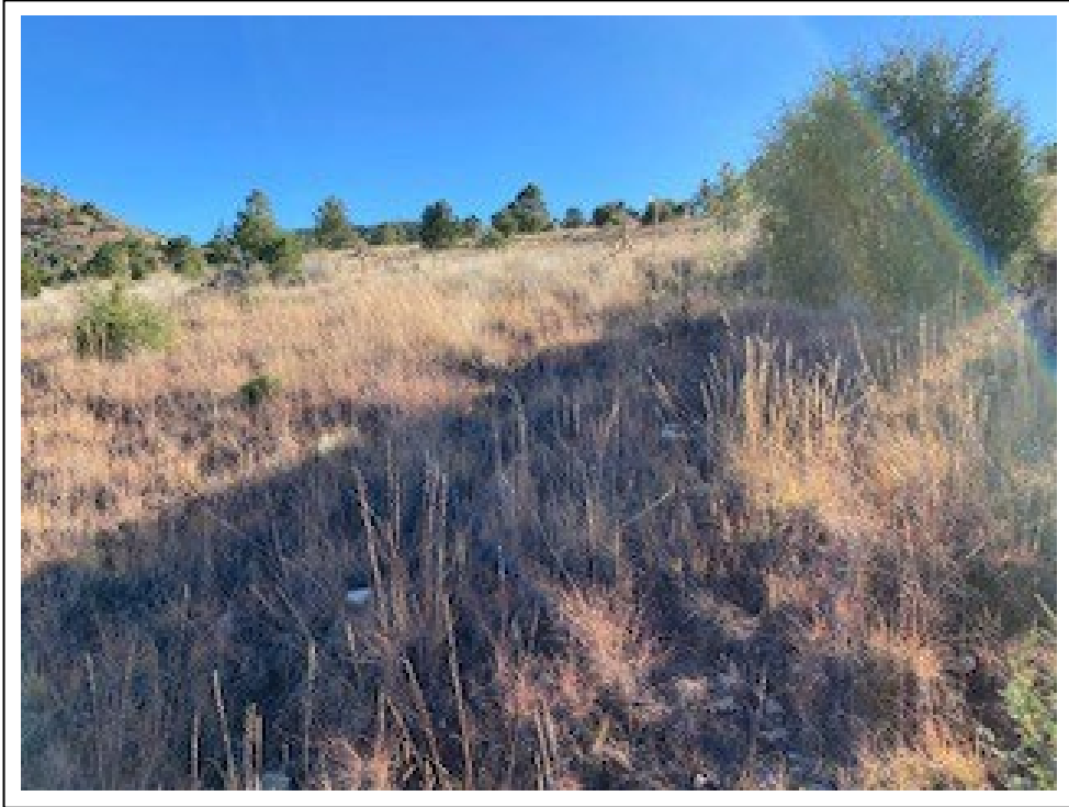
21. WRP location 11 prior to completion of repairs
