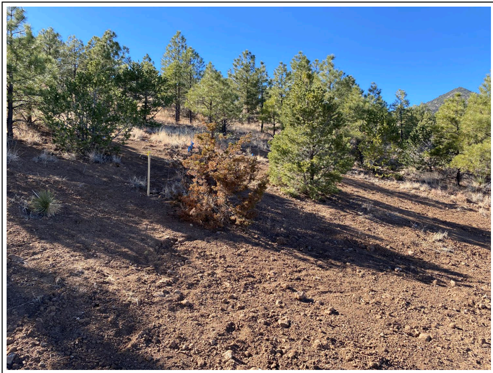
6. WRP location 3 after completion of repairs
