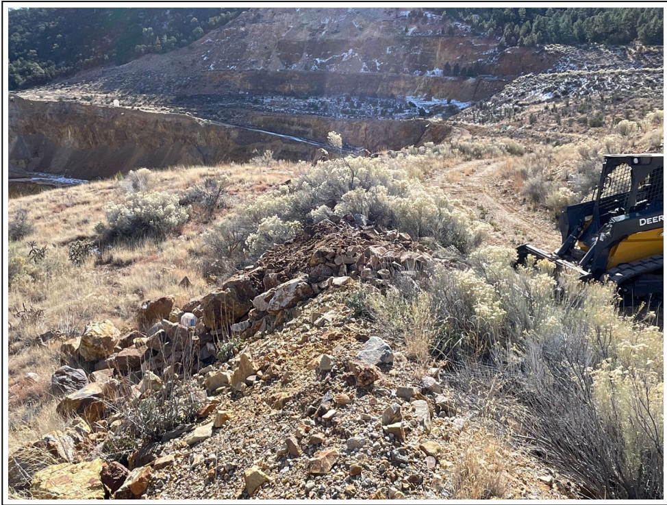
26. Pile of rocks (larger than 4 inches) removed
