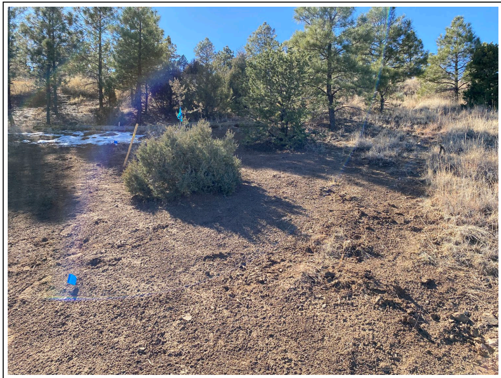
4. WRP location 2 after completion of repairs
