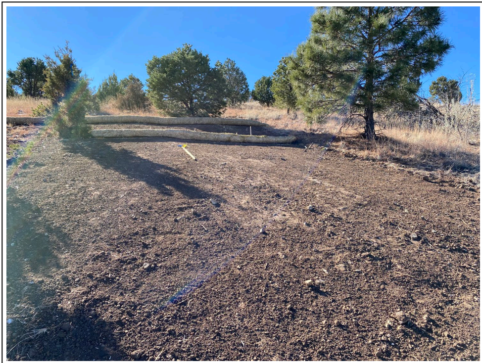
16. WRP location 8 after completion of repairs
