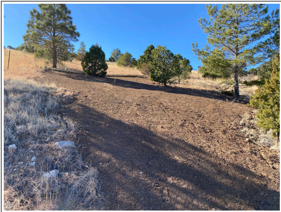
18. WRP location 9 after completion of repairs
