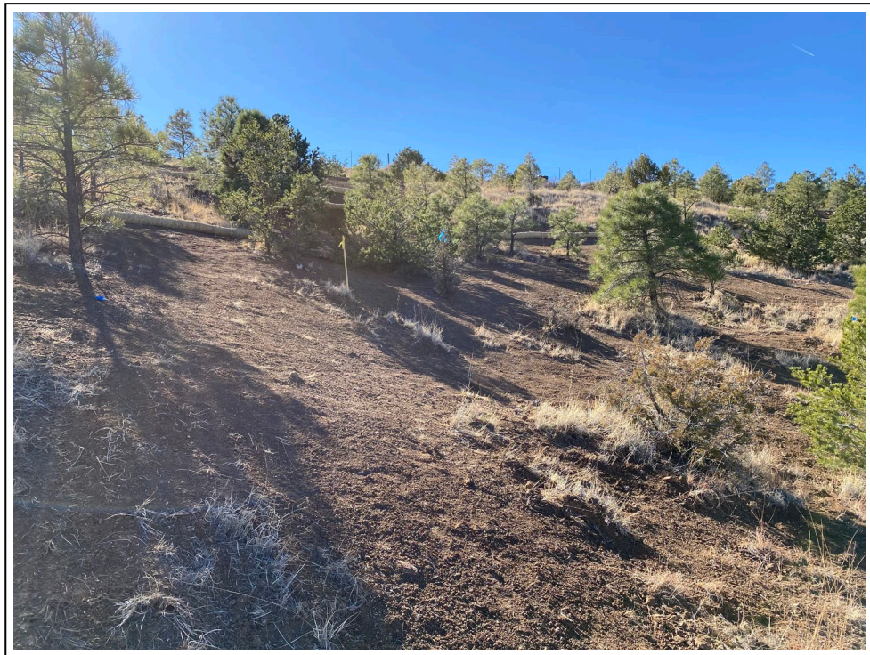
12. WRP location 6 after completion of repairs
