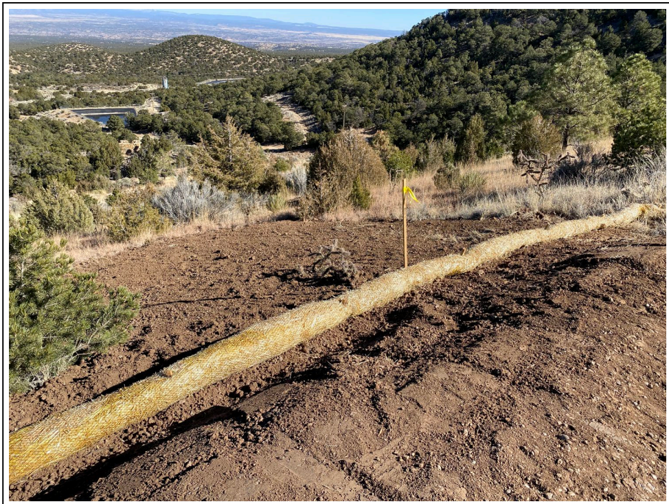
22. WRP location 11 after completion of repairs
