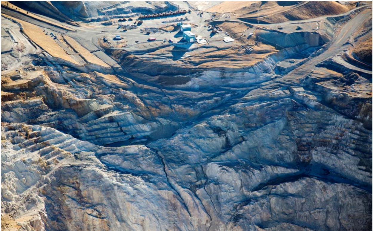
Figure 3. Montana Tunnels Pit Highwall Instabilities. (Photo by Christopher Boyer)
