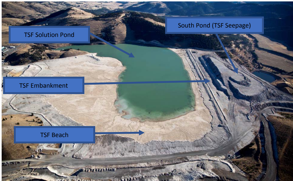
Figure 6. Montana Tunnels Tailings Storage Facility. (Photo by Christopher Boyer)
