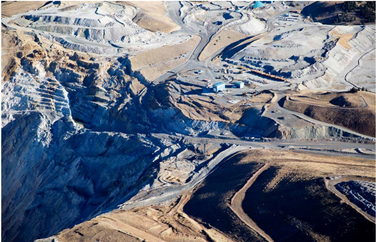
Figure 4. Montana Tunnels Pit Entrance and Access Ramp. (Photo by Christopher Boyer)
