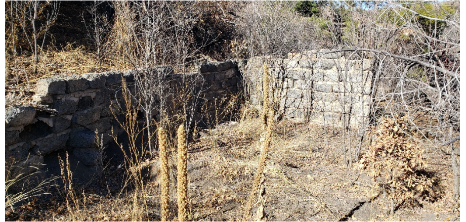
Photo 20. Mine structures by Adit A-3.
