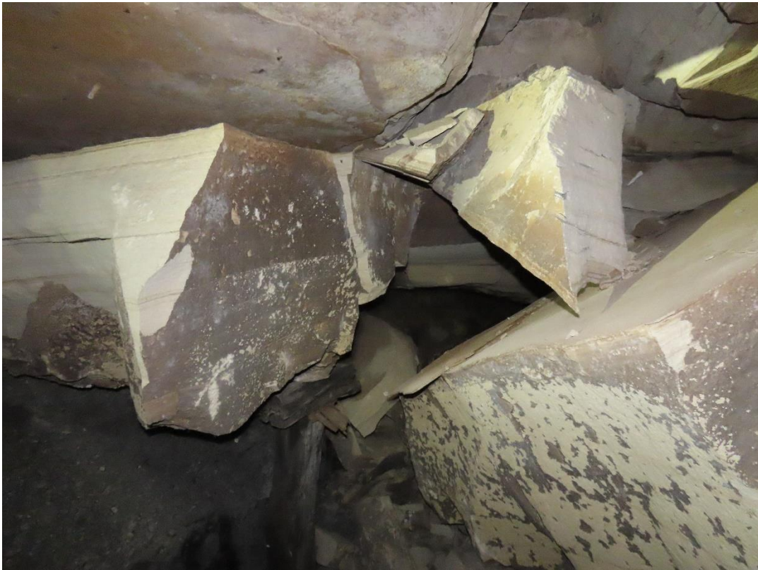
Yankee Adit 02: Another view of the dangerous blockage.
