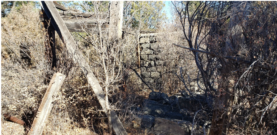
Photo 19. Mine structures near Adit A-3.
