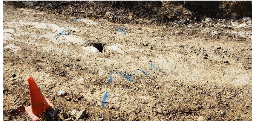
Photo 14. GPRS marking scans made with GPR units.
