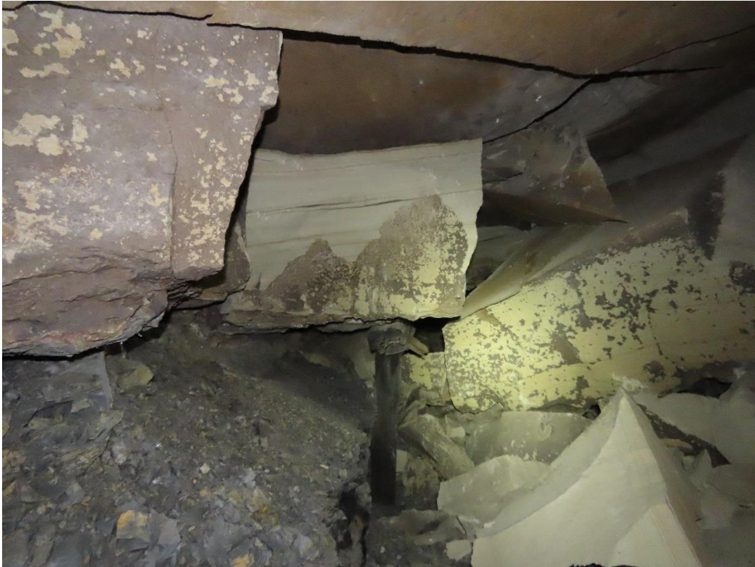
Yankee Adit 02: The dangerous section that prohibited passage. Note the large, rectangular white block balanced on a single old timber stull.
