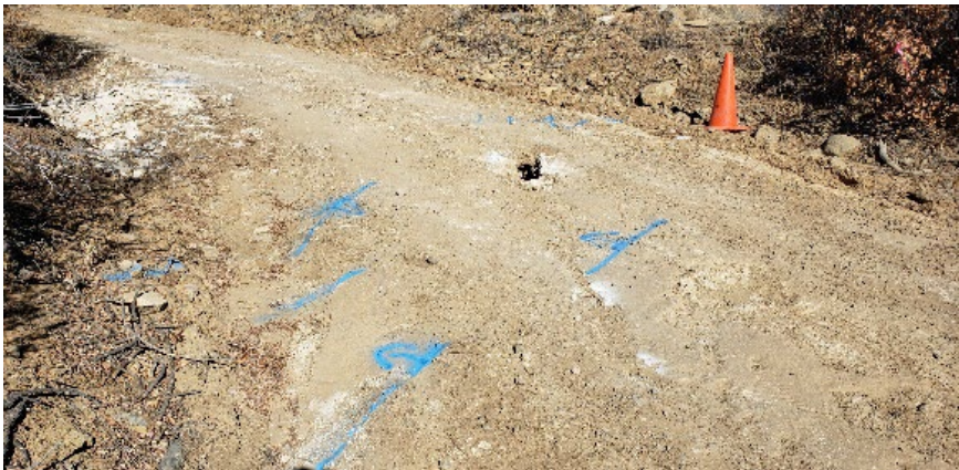
Photo 15. GPRS marking scans made with GPR units.
