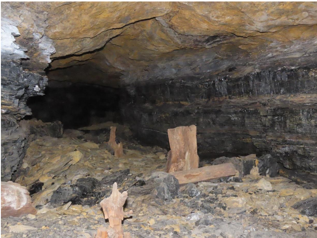
Yankee Adit 01: The coal seam is visible along the ribs. BCI Photo by Bill Burger
