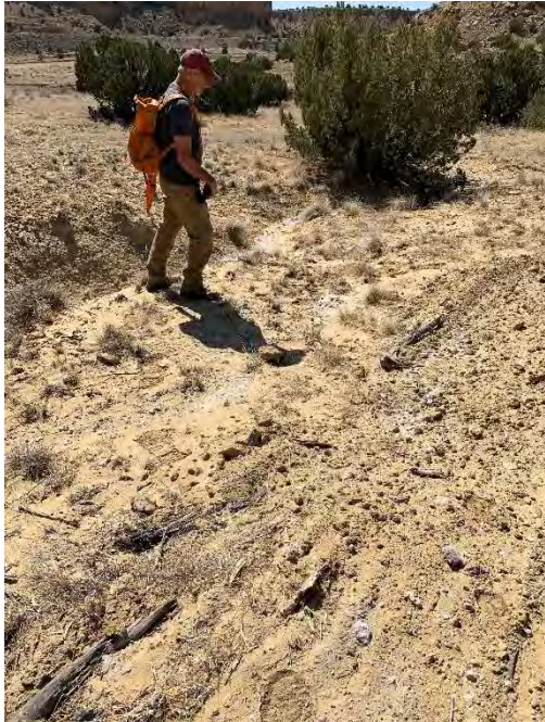
FIGURE 16 ENTRY OF FLOW INTO THE DRAINAGE OFF DRILL PAD A8
