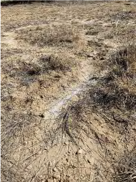
FIGURE 15 MUD DRAINING DOWN AWAY FROM DRILLPAD TO THE ROAD (A27)
