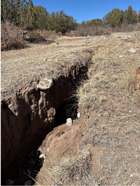
FIGURE 52 HEADCUT IN THE ROAD - PREVIOUSLY NOTED IN PRIOR INSPECTION (2016)
