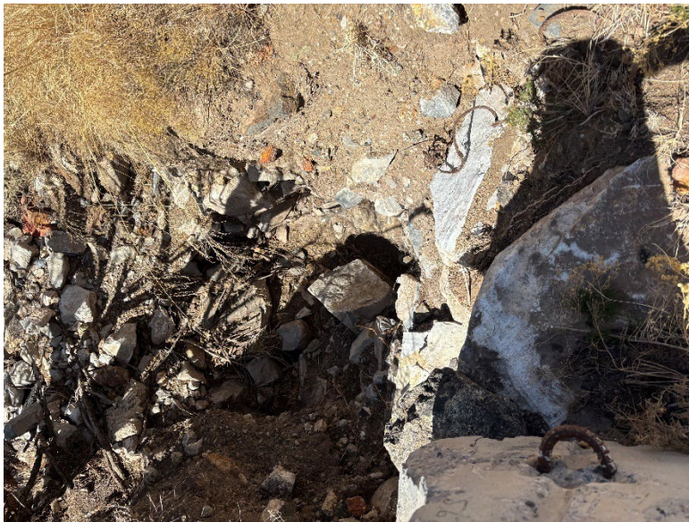
FIGURE 51 CEMENT BARRIER VISIBLE IN THE BOTTOM, DIRT AND ROCKS ARE WASHED OUT FROM UNDER THE BARRIER.
