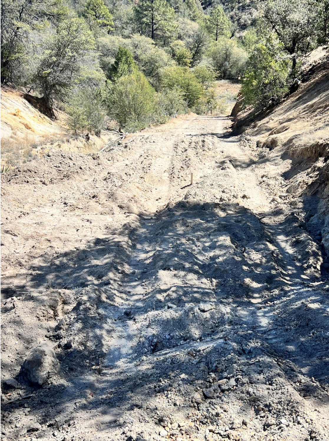
Permitted hole #8, Sugarloaf drilled hole SL-2. Pad dimension of 14' x 52' - 36% of permitted disturbance. The remainder of the pad utilized the road as passability was not an issue.
