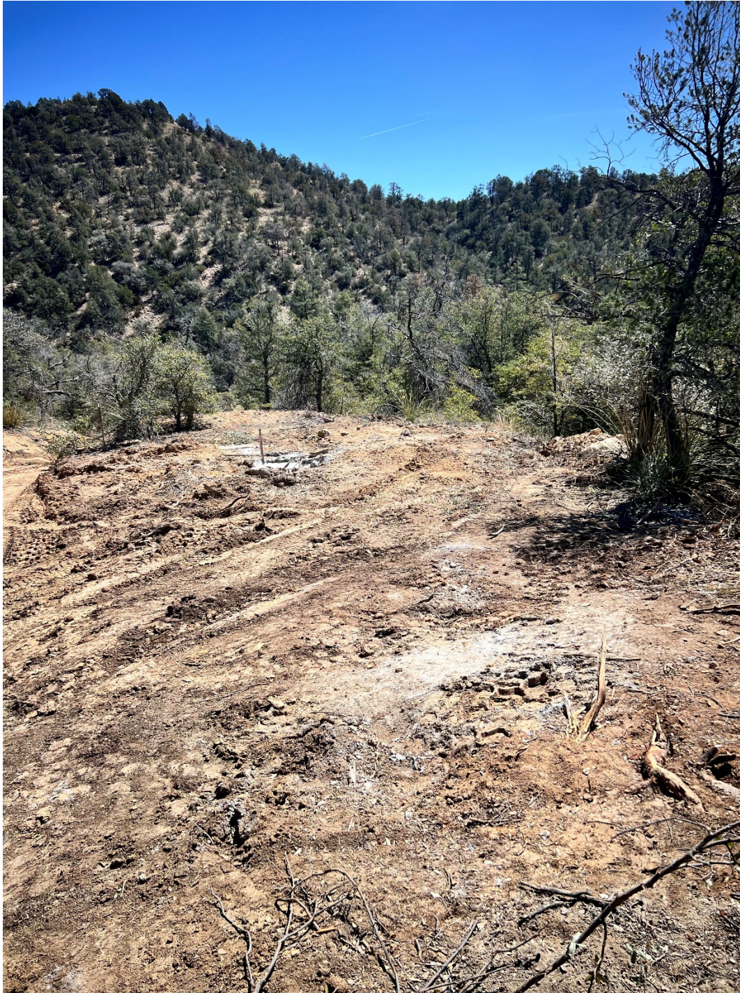
Permitted hole #7, Sugarloaf drilled hole SL-4. Pad dimension of 20 x 78' - 78% of permitted disturbance.
