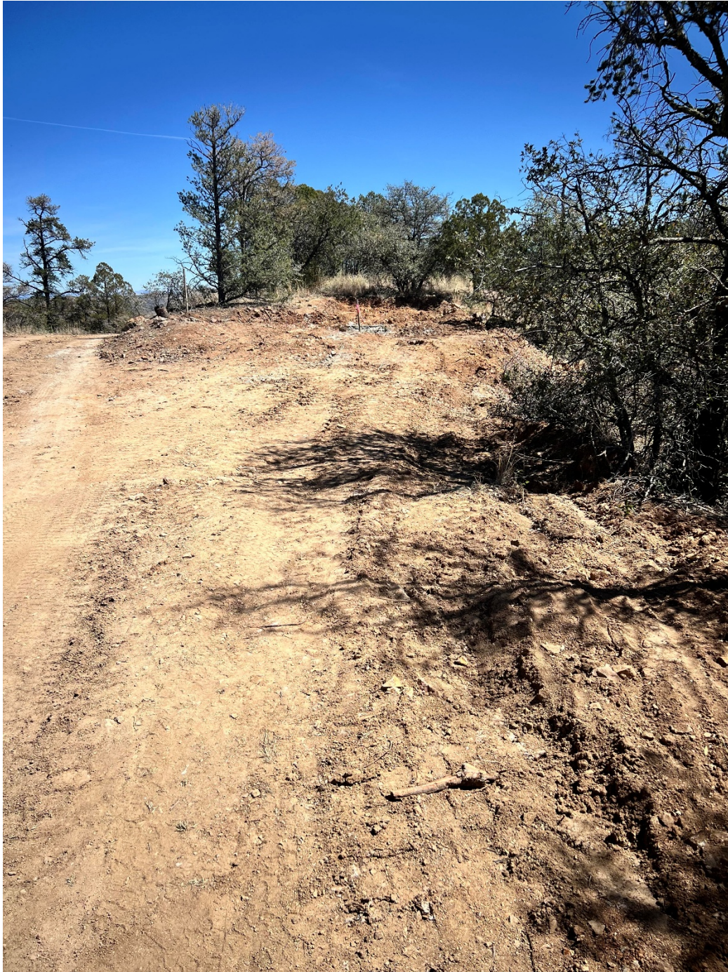
Permitted hole #6, Sugarloaf drilled hole SL-5. Pad dimension of 21' x 50' - 51% of permitted disturbance.
