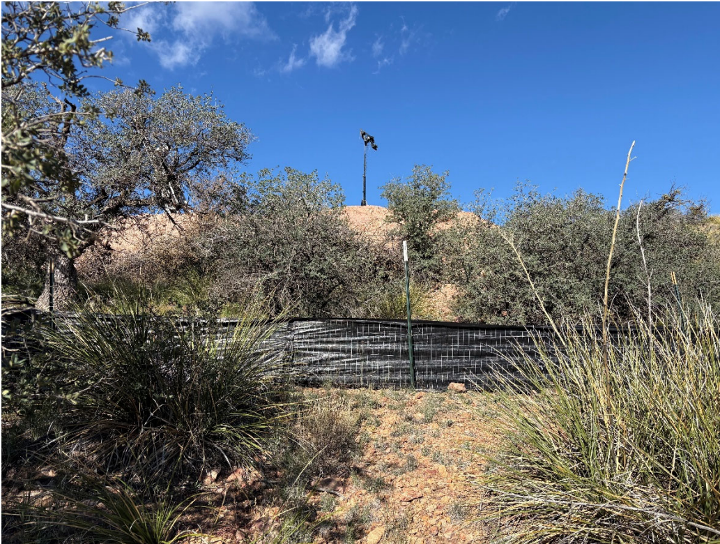
Image 7. Silt fences that will remain in place downgradient of open drill pads.
