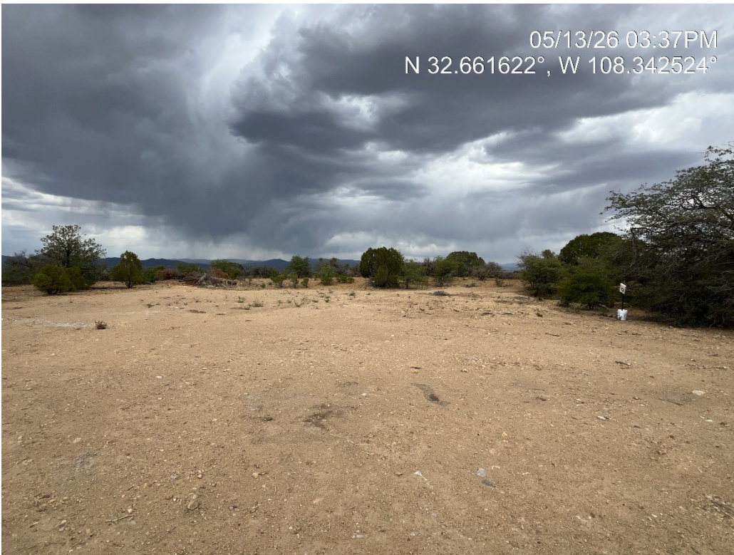
Image 4. Pad Q status after drilling was completed and the sump was backfilled.
