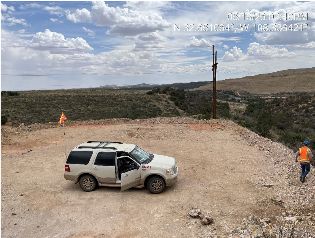
Image 1. Pad K status after drilling was completed and the sump was backfilled.
