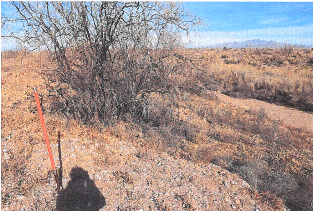
Repeat photo from November 2018. Tailings were removed and buried on the interior of the facility to prevent mobilization into the Mimbres River. Additional cover material was also applied to prevent additional erosion.
