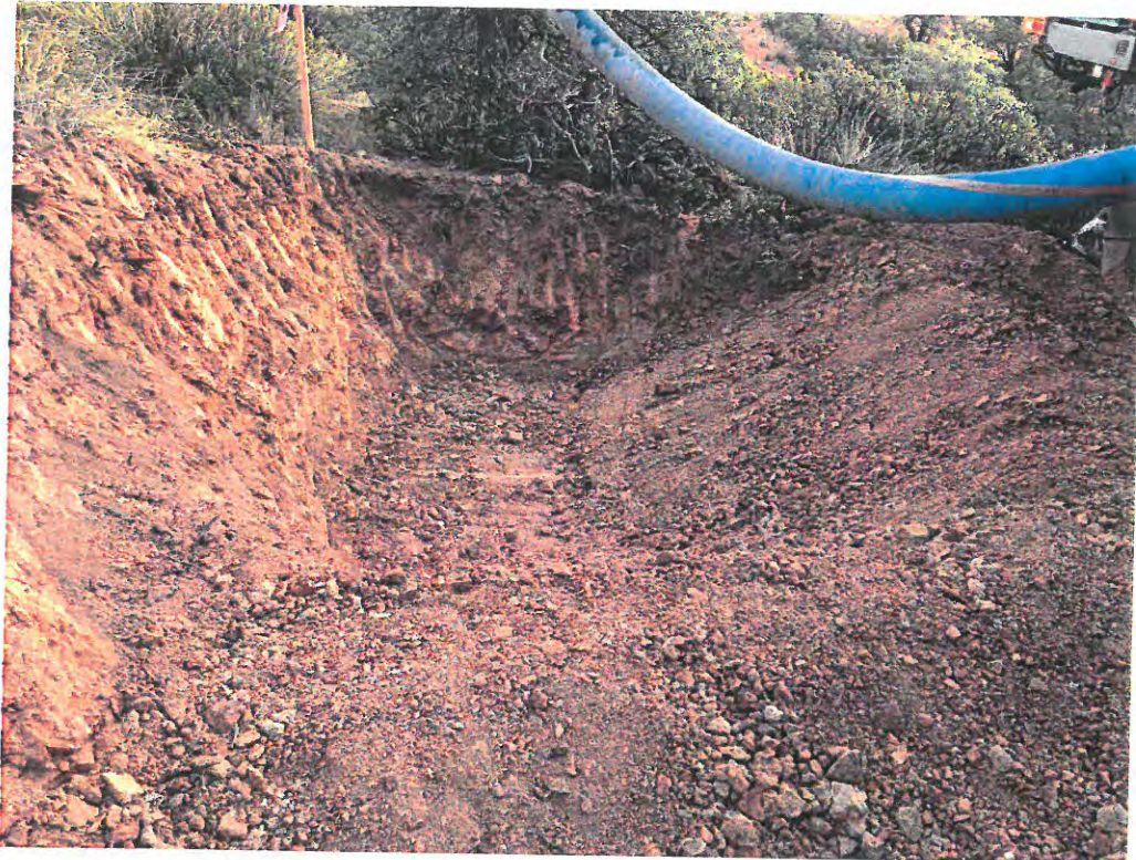
Photo 5: Excavated Sump for Drill Site 16, 8/22/18
