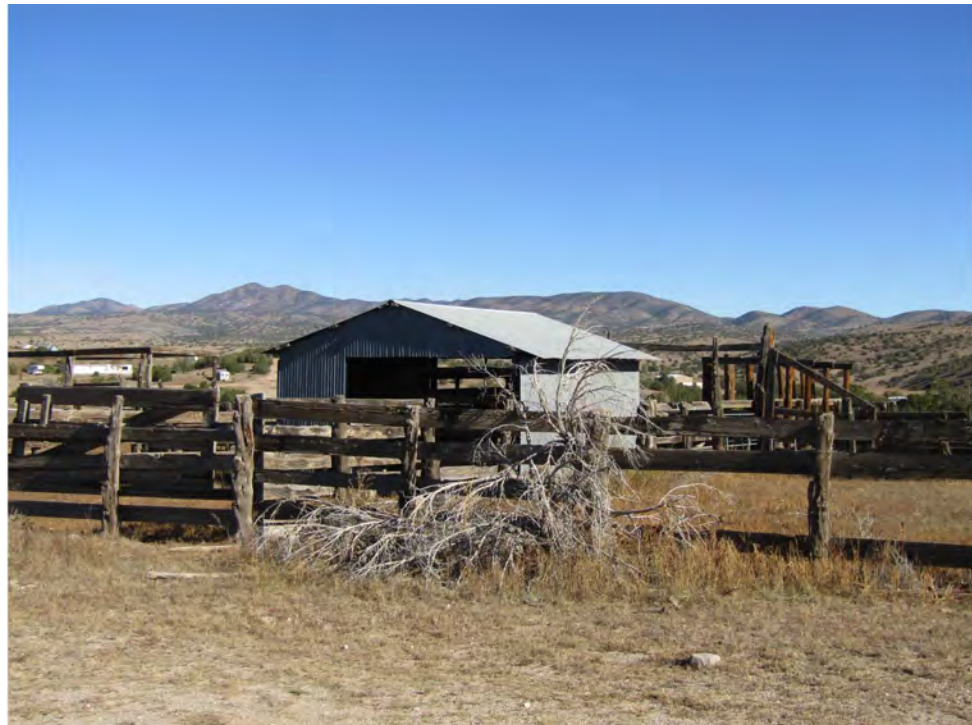
BELOW: View of livestock shed
