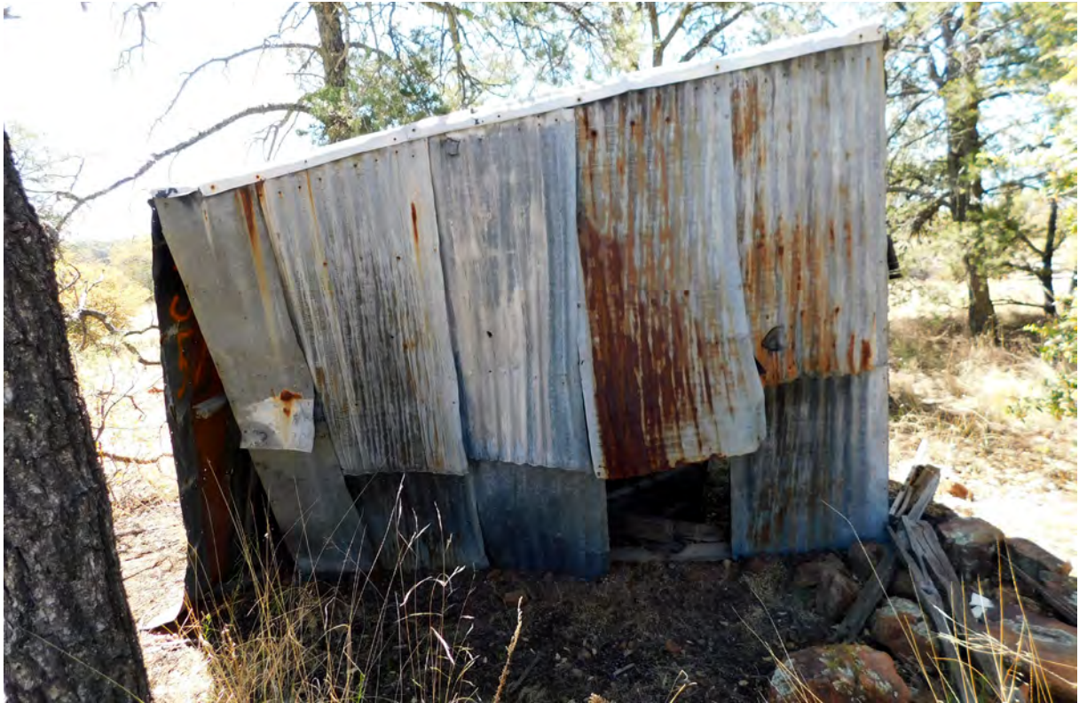
Photograph 18. AR 03-06-07-0669/LA 167143 Feature 1 (Rear View)
