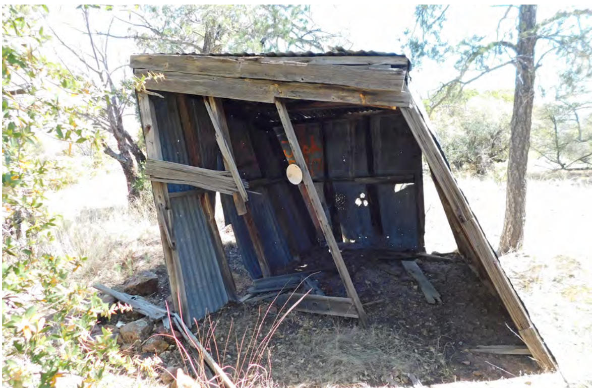
Photograph 17. AR 03-06-07-0669/LA 167143 Feature 1 (Wood and Metal Shed) from the Front
