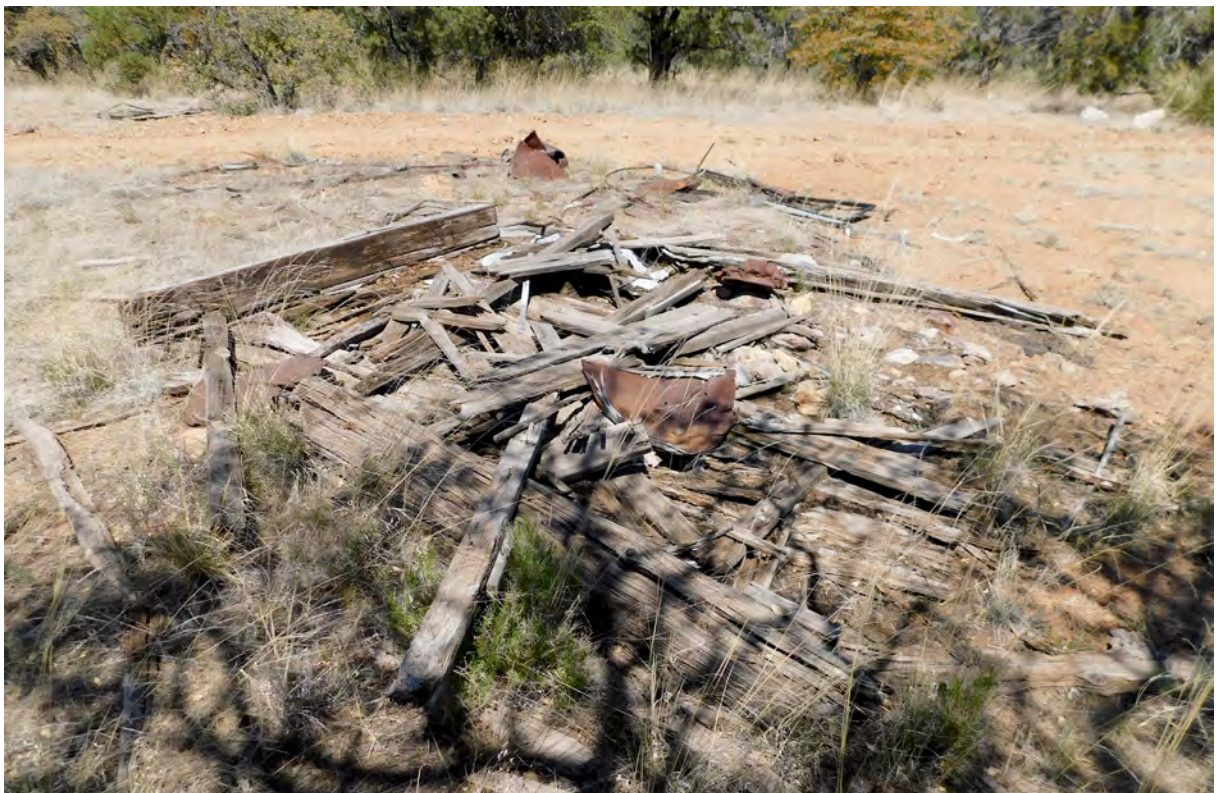
Photograph 19. AR 03-06-07-0669/LA 167143 Feature 3 (Collapsed Wooden Structure)
