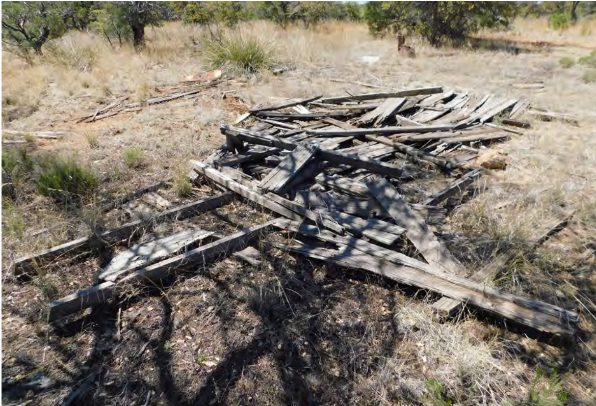
Photograph 20. AR 03-06-07-0669/LA 167143 Feature 4 (Collapsed Wooden Structure)
