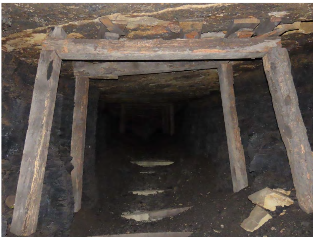
NEW Black Rose Mine-SW_ SP-3 S. Subsidence 1: Historical timber supports in the main drift. BCI Photo by Dillon Metcalfe
