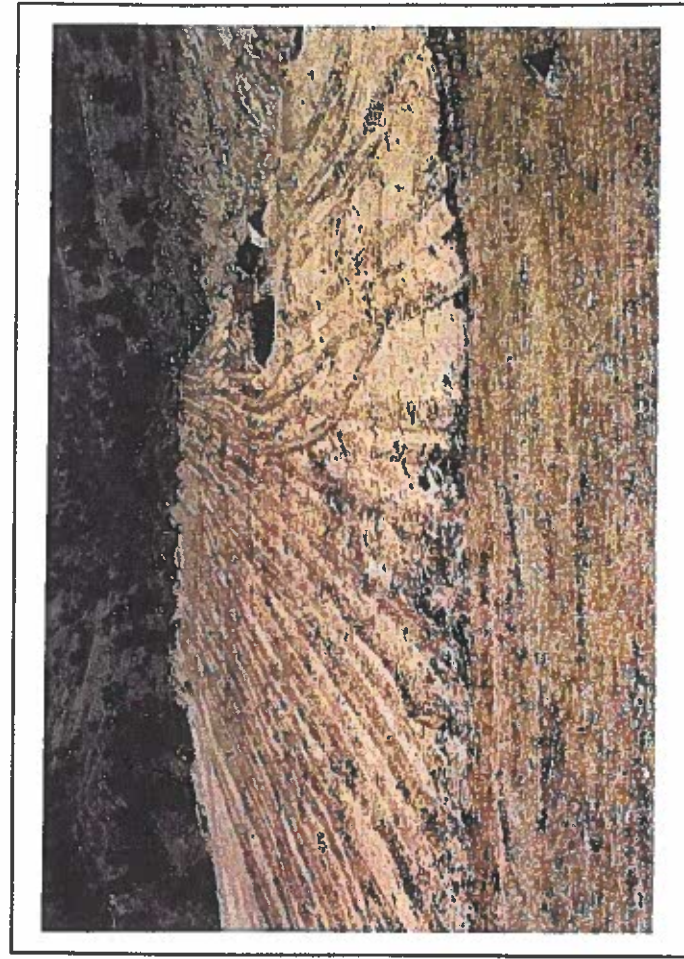
Figure 19 Track Walking of Slopes - Erosion Control
