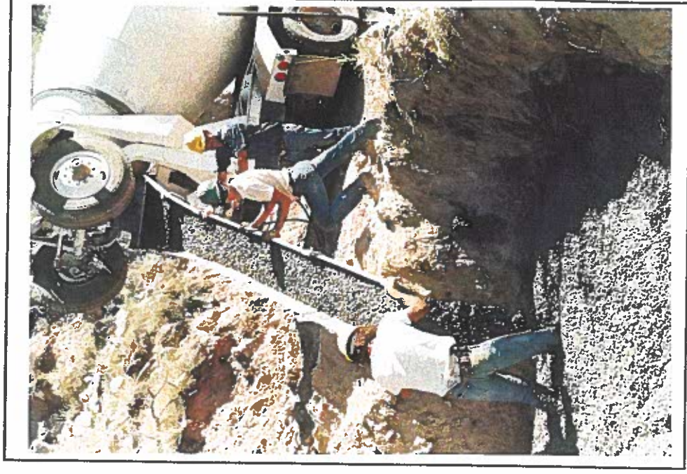
Figure 15 Cement Cap at Vent Raise
