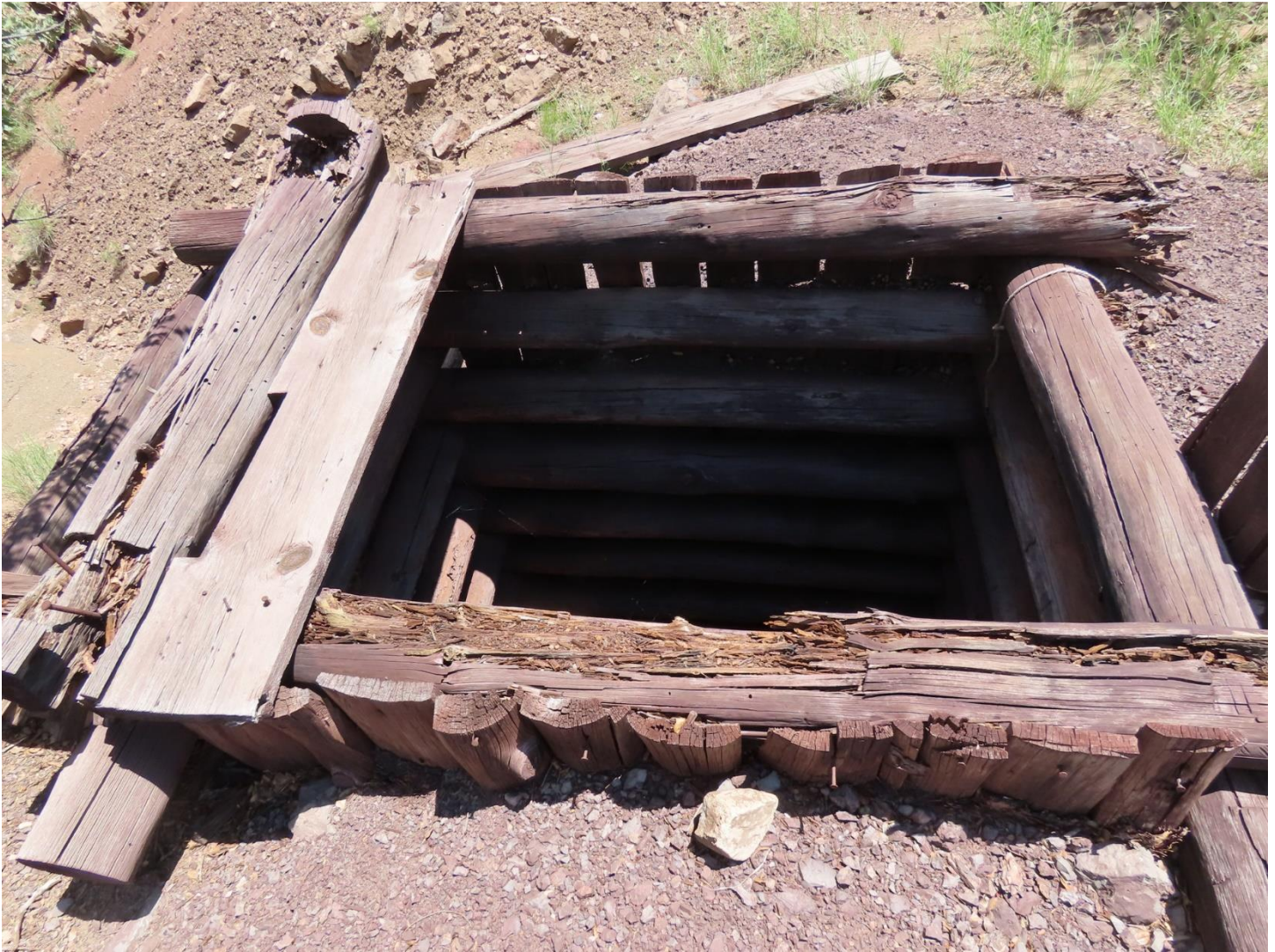
Homick Energy Maggie Mine Shaft: Sturdy timbers support the collar of this mine shaft.
