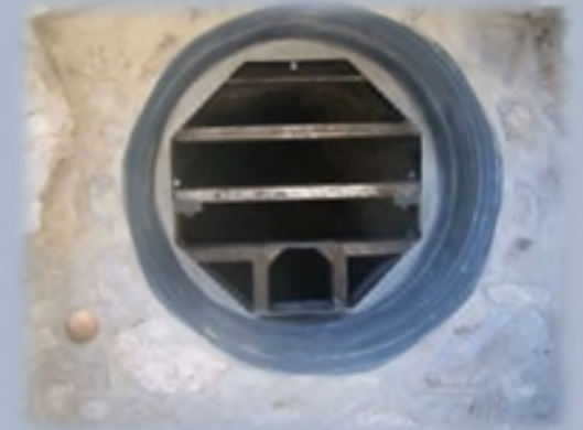
Bat Gate in Rock Bulkhead
