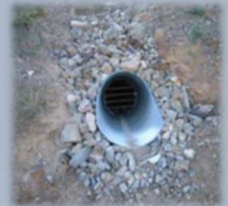
Culvert with Bat Gate
