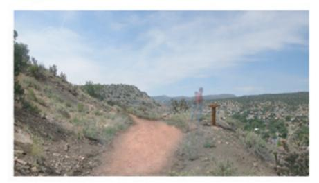
After - Improvements to the trail include removing excess vegetation and using 'red dog' for trail stabilization. Interpretive signage could be added at appropriate locations.
