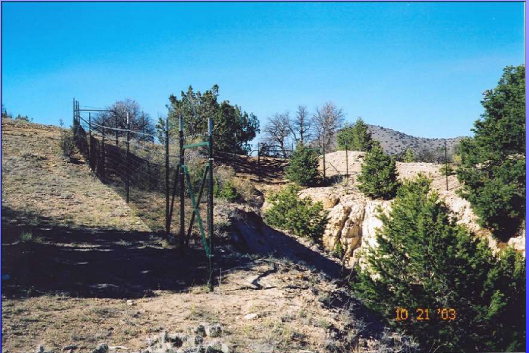
Wire Mesh Fence at Trench Highwall
