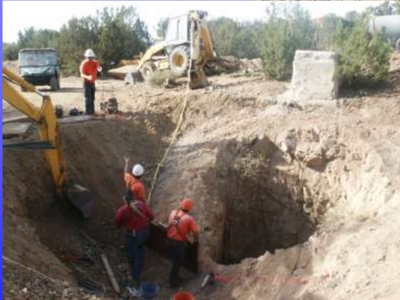
Concrete Collar with Wire Mesh At Mina del Tiro
