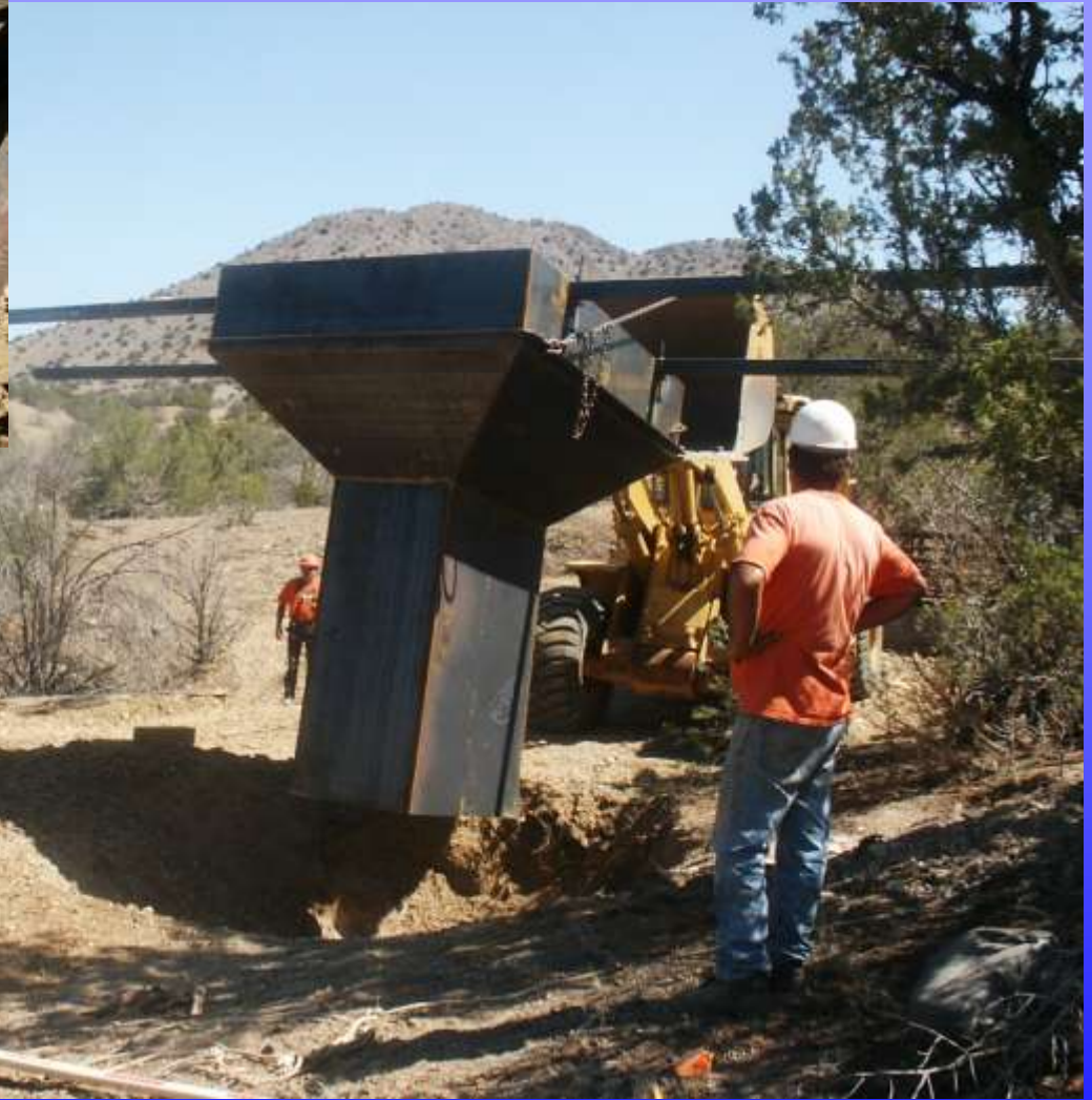
Installing Structural Tubes for Bat Cupolas
