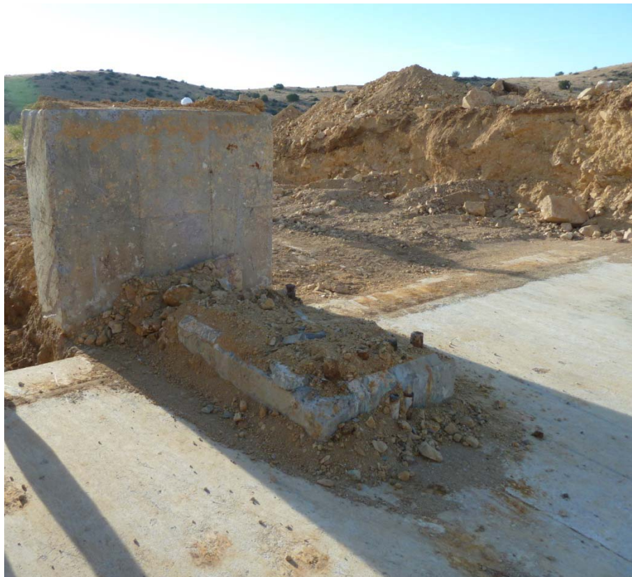
Photo 14 – Typical Column Base at E3
