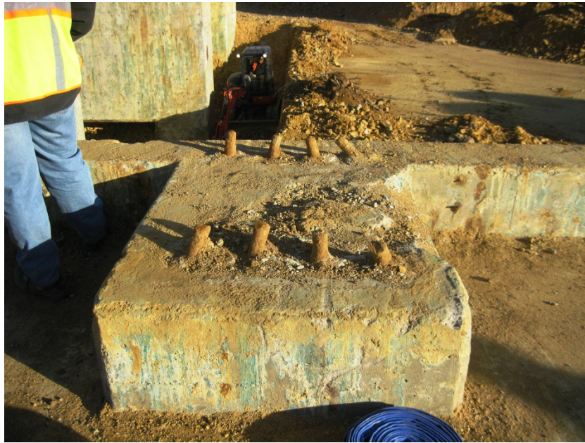
Photo 11 – Concentrator – Typical Building Pier
