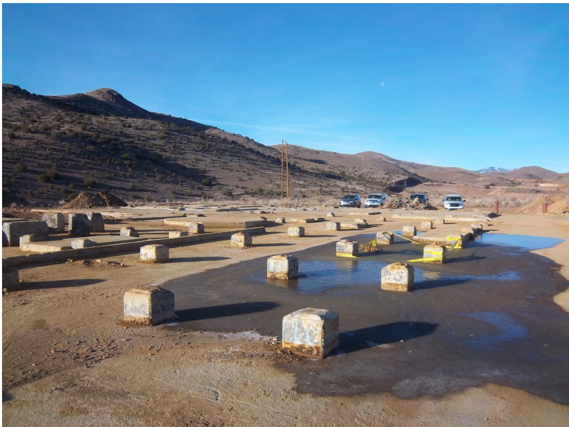
Photo 8 – Flotation Area – Existing Interior Concrete Piers
