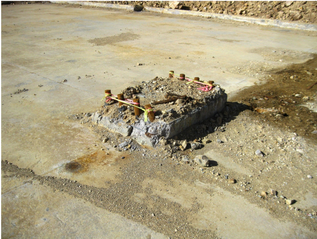
Photo 13 – Truck Shop – Spalled Concrete, Exposed Rebar and Corroded Anchors at Interior Concrete Pier
