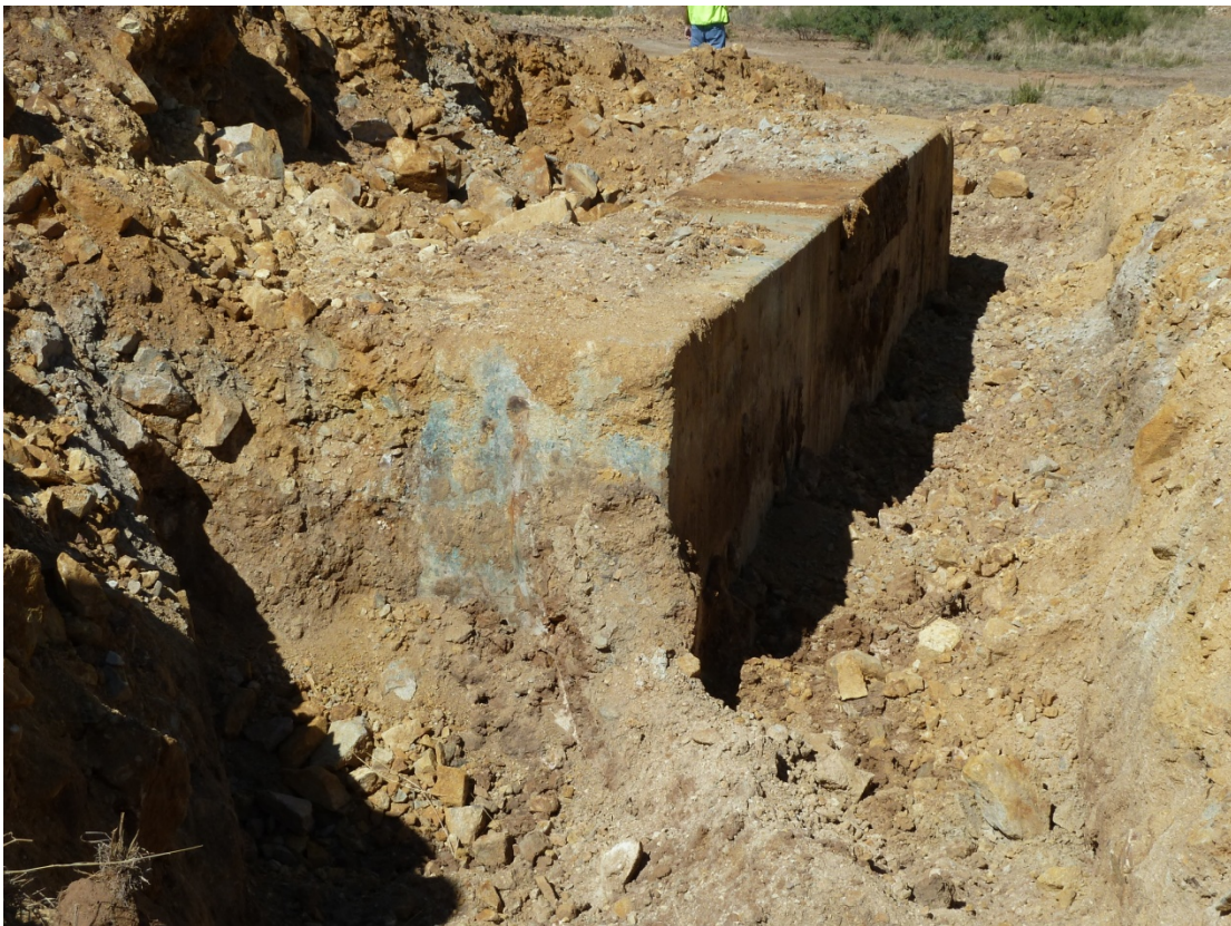
Photo 4 – Primary Crusher Dump Pocket
