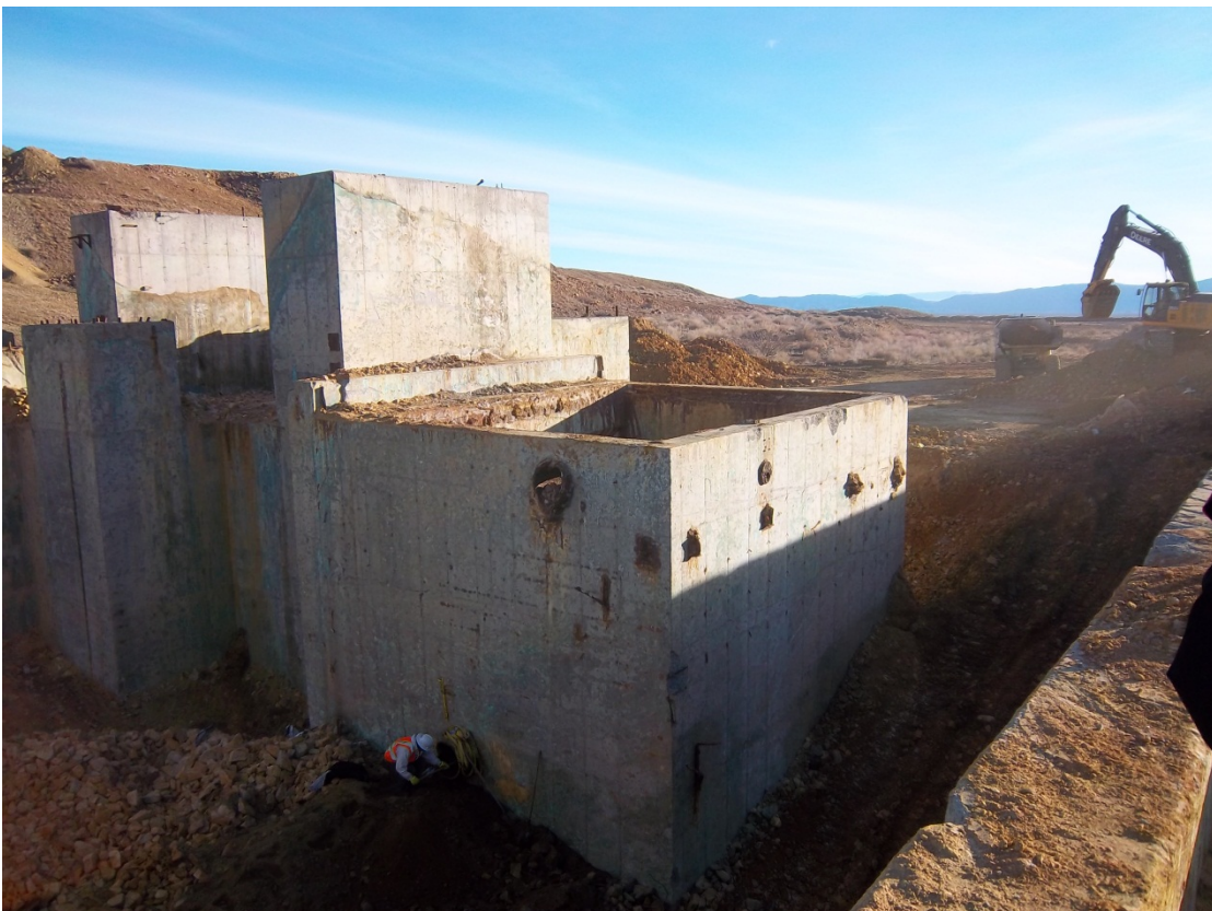
Photo 10 – Grinding Area – Corroded Embeds at Sump Box
