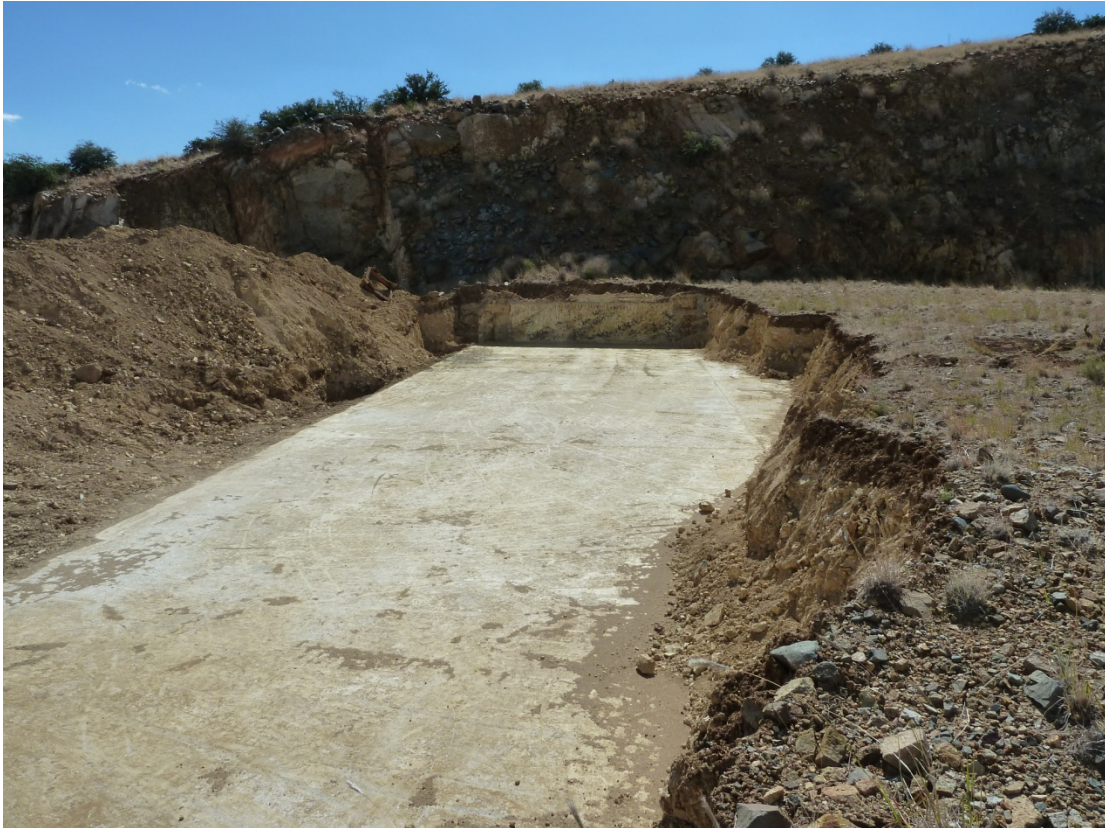
Photo 19 – Concentrator Stockpile With Push Wall at Rear
