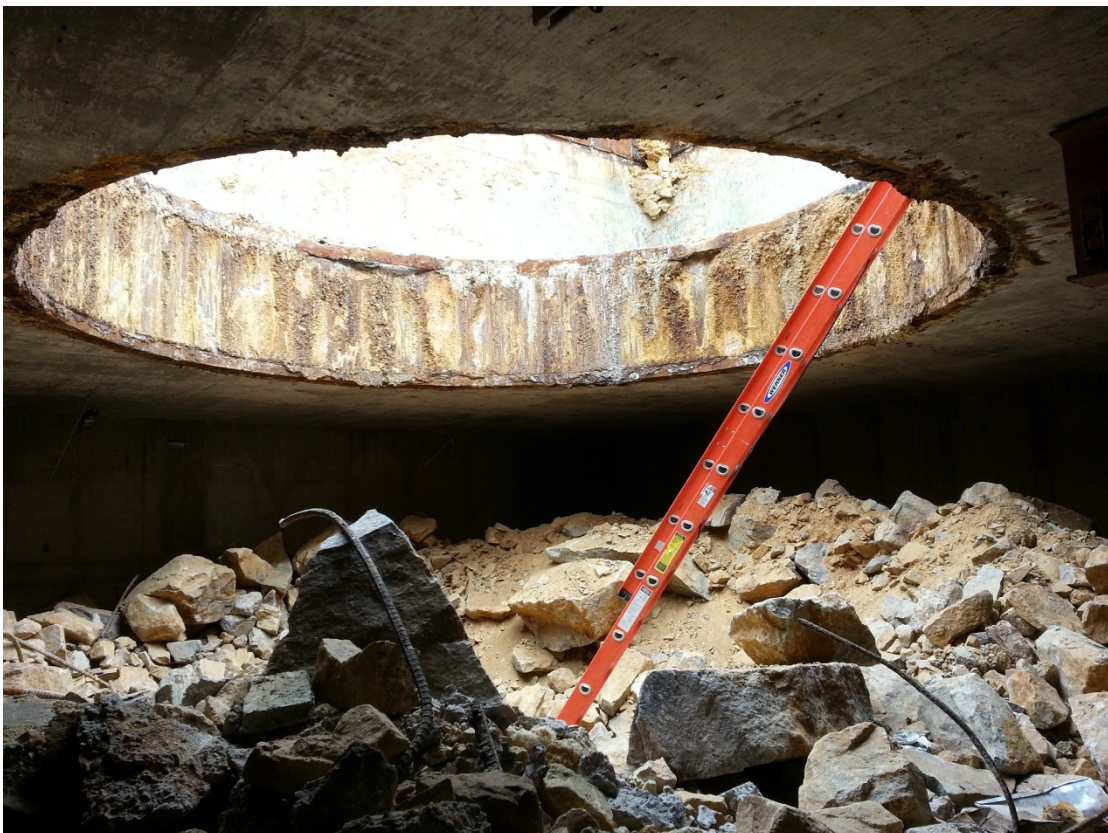
Photo 4 – Primary Crusher – Corrosion on Embedded Items
