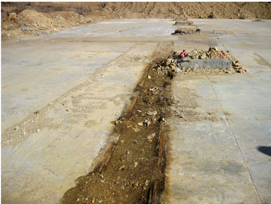
Photo 14 – Truck Shop – Corroded Electrical Trench Embed Angle
