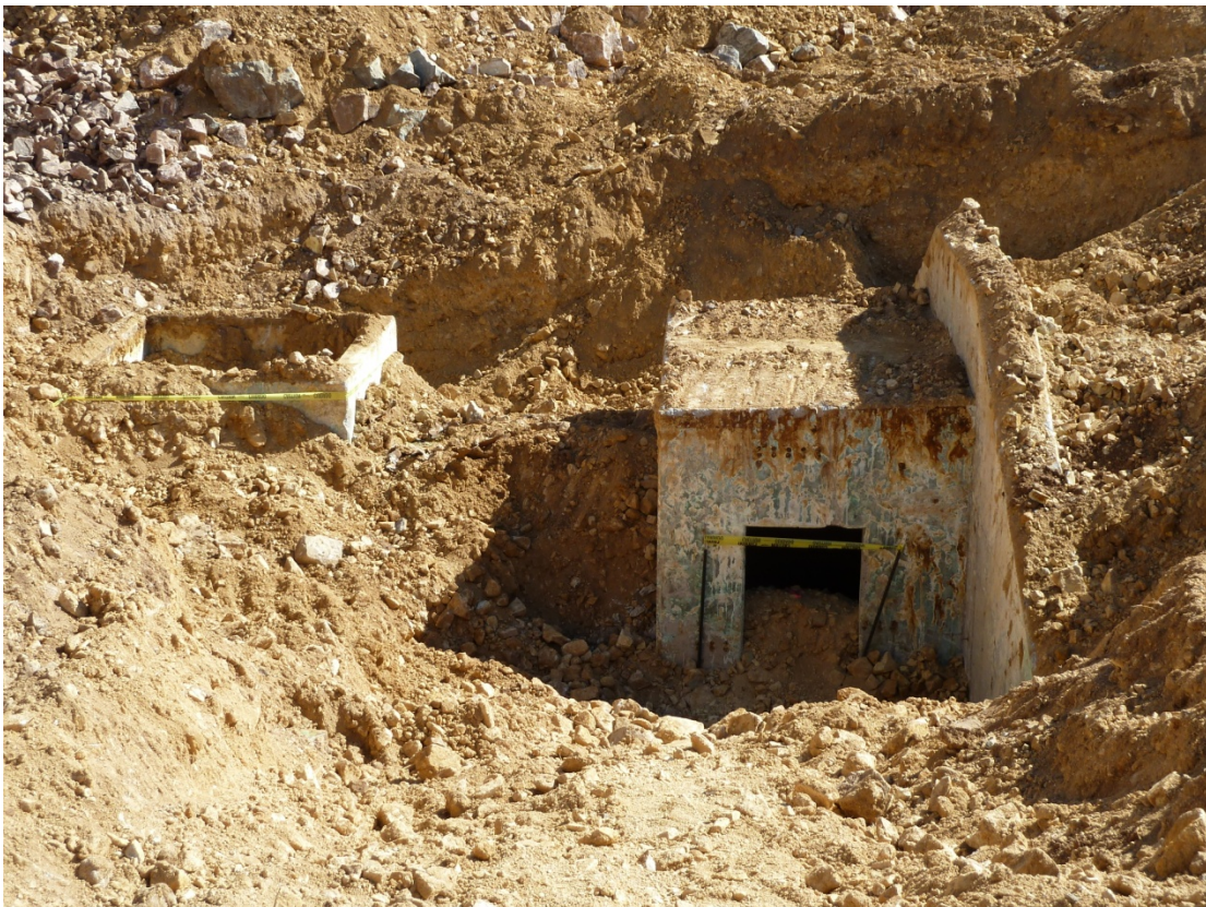
Photo 10 – Reclaim Tunnel Escape Manway and Valve Box
