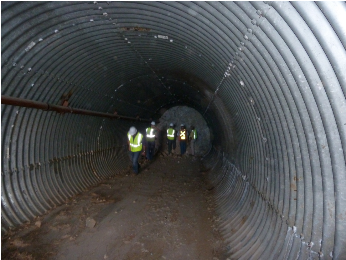
Photo 3 – Multiplate Tunnel
