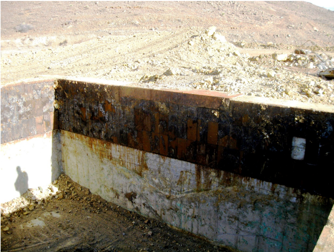
Photo 3 – Primary Crusher – Greenish-blue Discoloration at Wall Surface
