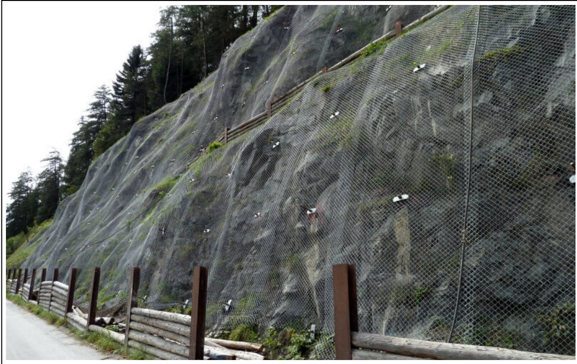
17. Spyder mesh: Steel mesh constructed of braided strands of high tensile strength steel wire
