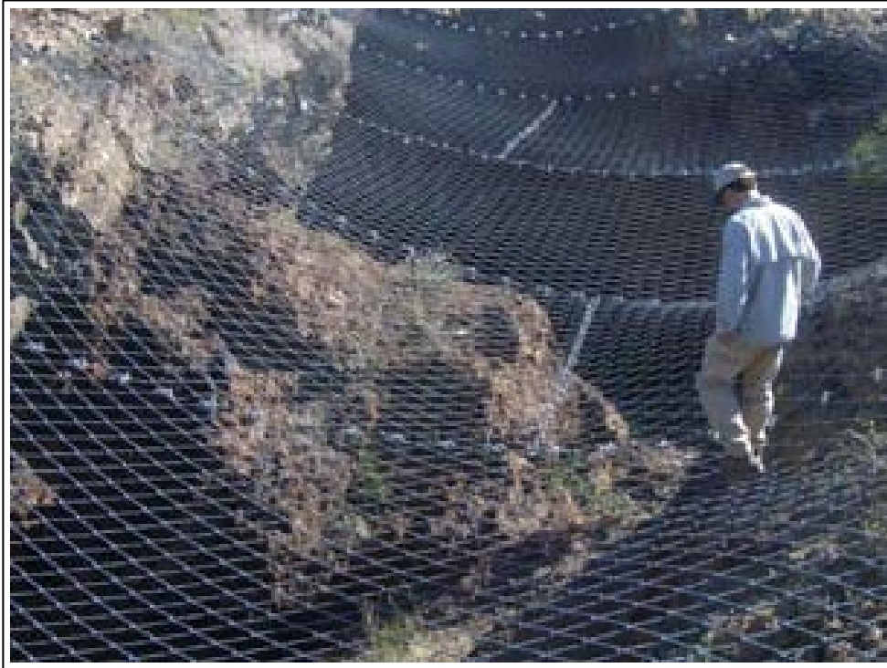
15. Spyder mesh: Steel mesh constructed of braided strands of high tensile strength steel wire
