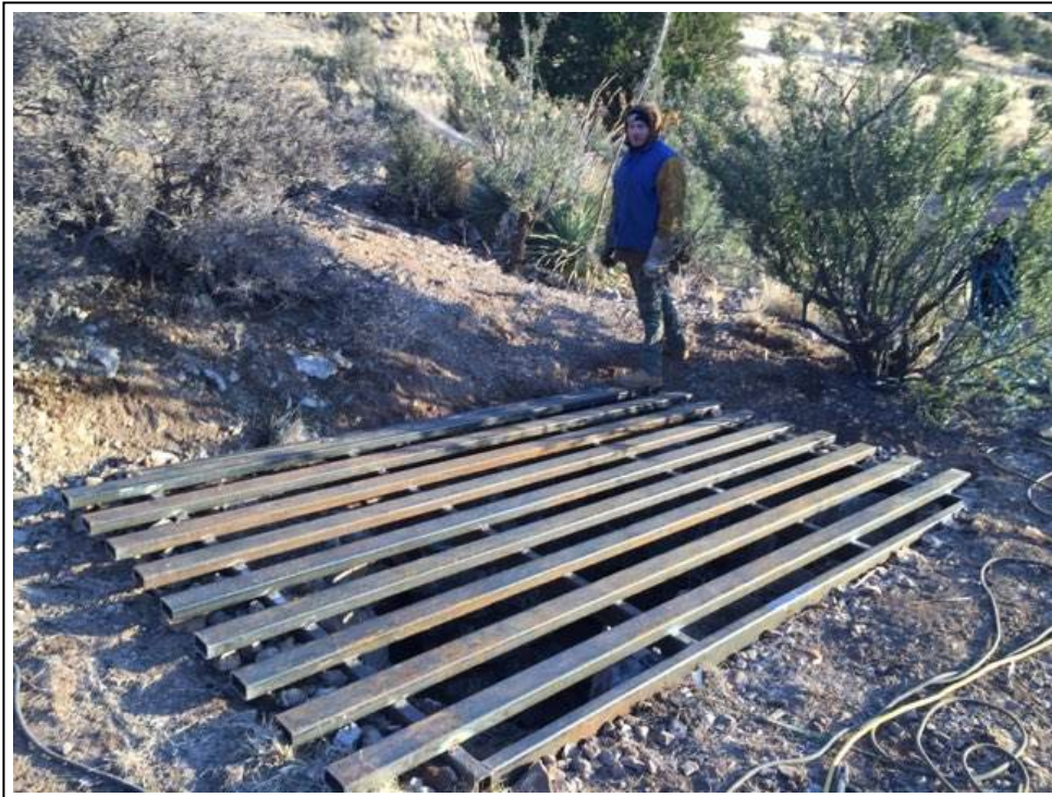
9. Example of steel gate for vertical shafts
