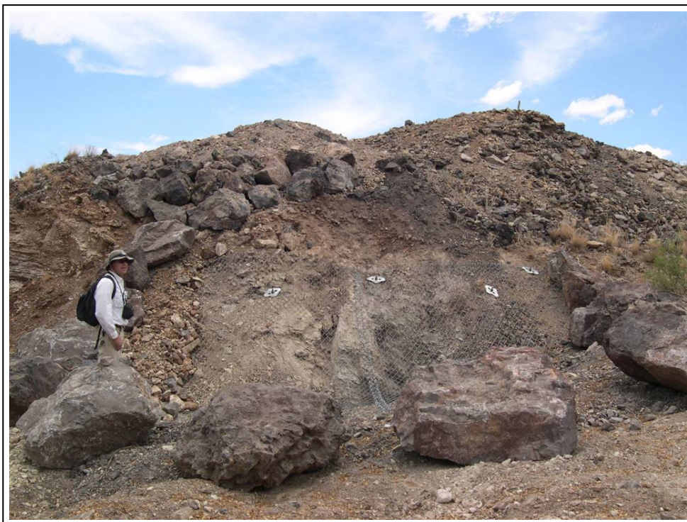
10. Example of Spyder steel mesh panel over shaft
