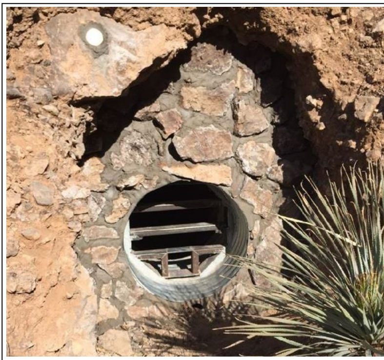
12. Example of a rock/concrete bulkhead with culvert gate
