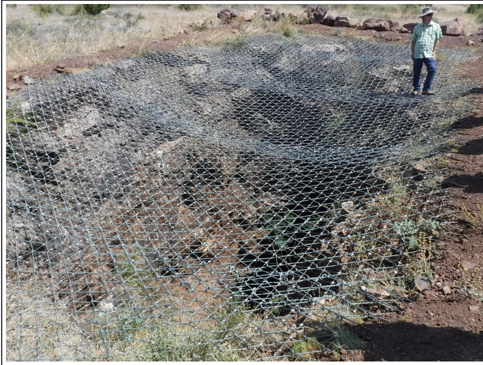
7. Southeast quadrant: Recently constructed wire mesh covering over open pit
