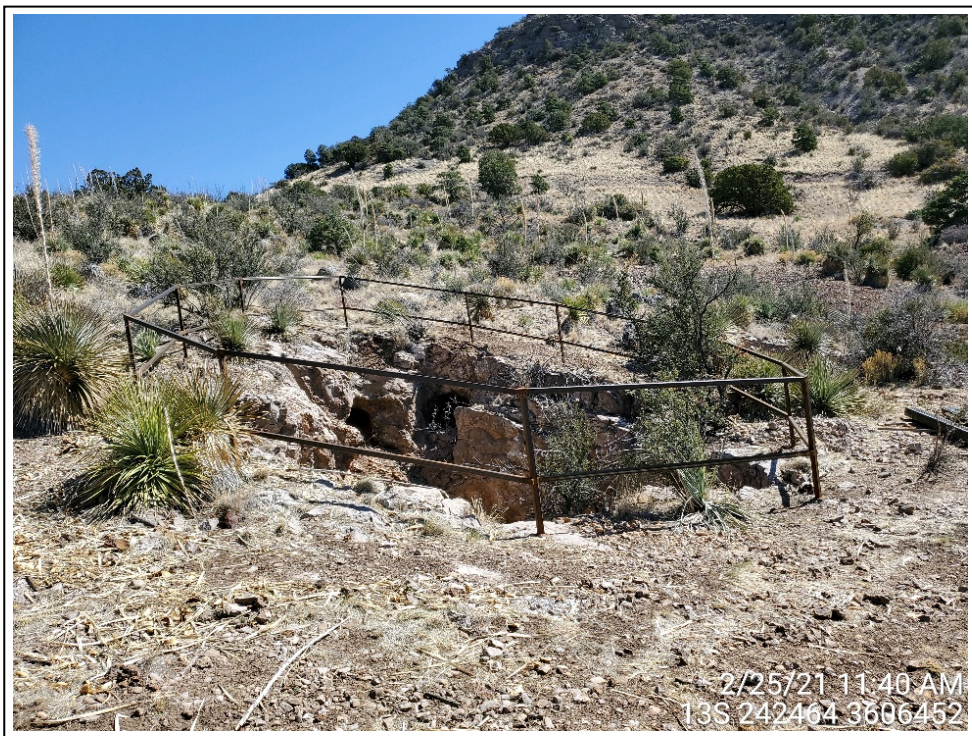
16. Tubular steel two-rail fence for high walls
