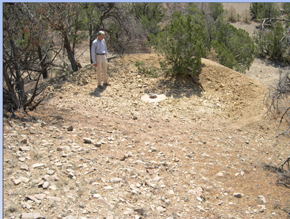
A complete polyurethane foam closure with beehive grate and concrete collar
