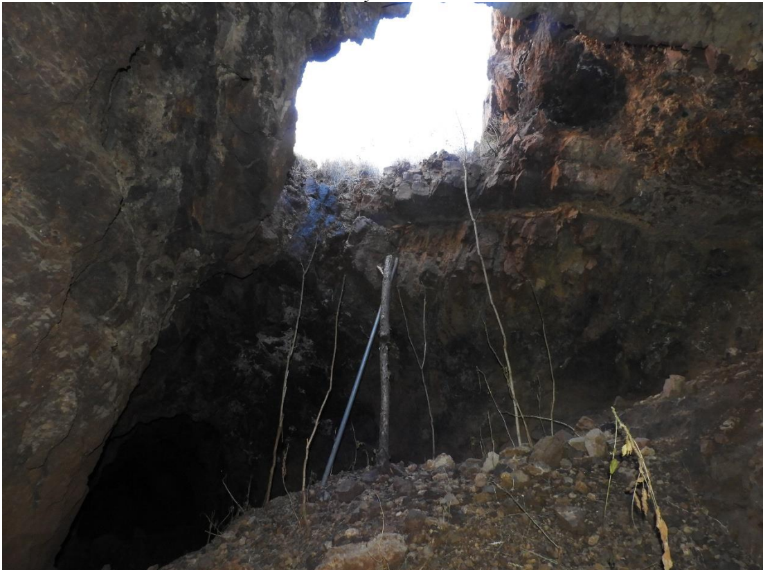
AMLCHLT18SR14WS03_39: Collapsed material lies below an opening in the lower workings.
