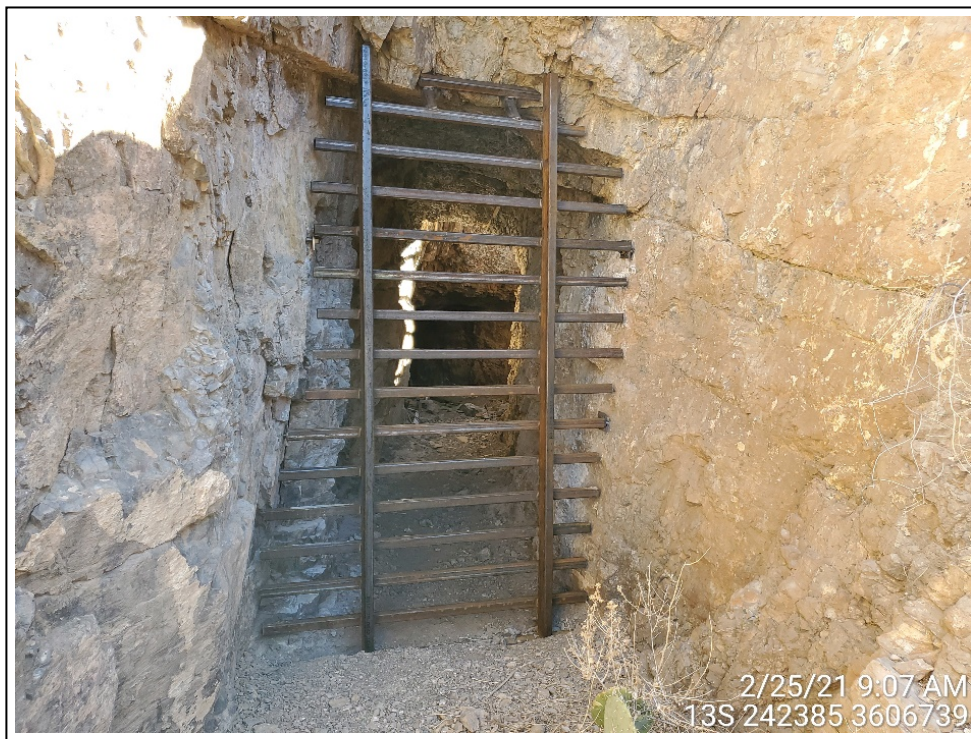
11. Example of steel gate over adit
