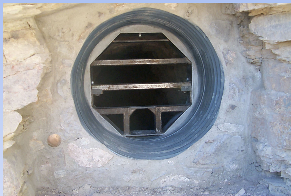
Culvert with bat and wildlife-friendly gate
