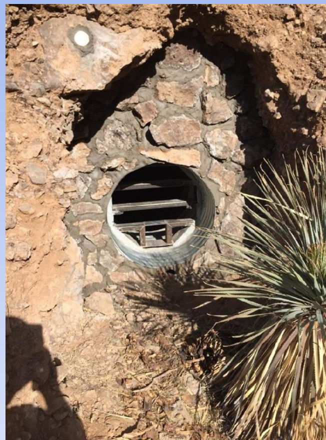
Rock bulk-headed culvert with bat-friendly gate. Cemented rocks assist with blending into landscape
