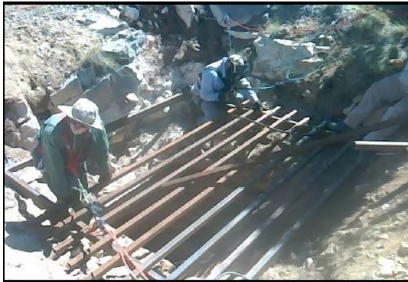
Installation of a bat gate.
