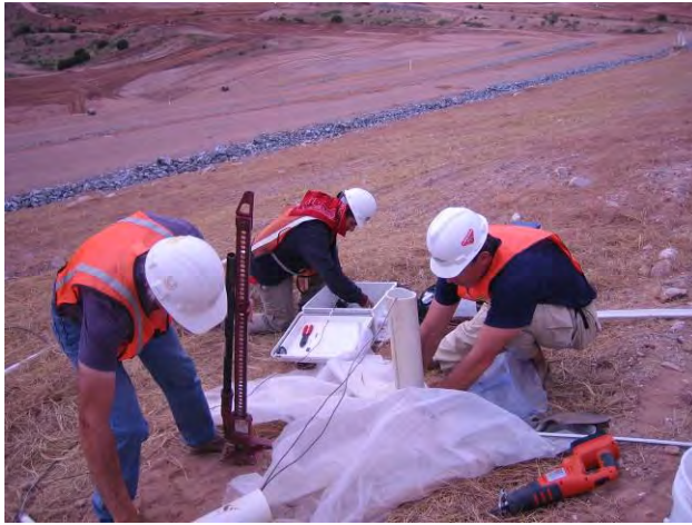
Down-hole HDS installation
