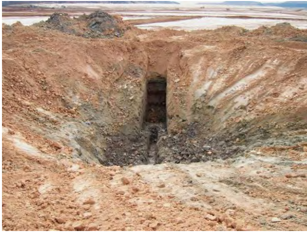
Excavation of 5B Lysimeter
