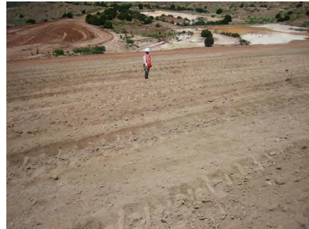
Outslope cover prior to scarification - May 05
