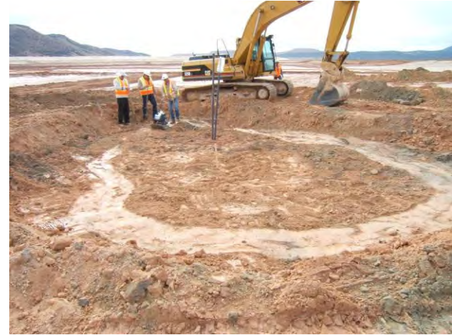
Lysimeter 5B backfill compaction
