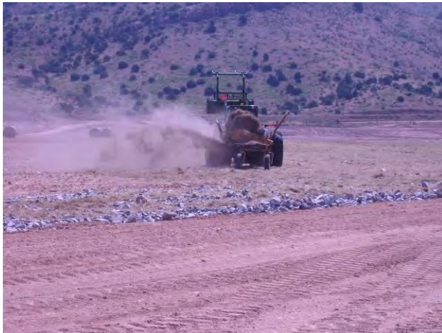
Spreading mulch – June 05
