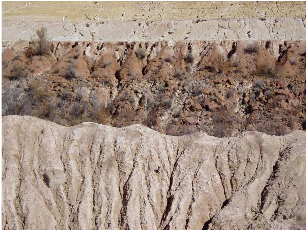
Figure B-7. Water deposited tailing (map unit 50) on the southwest face of the No. 2 starter dam. Tailing in foreground is contained by the catch basins below the starter dam.
