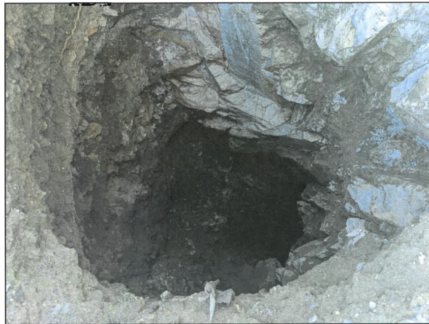
3 PHOTO OF SUB-2 LOCATION EXISTING CONDITIONS - LOOKING DOWN INTO OPENING
