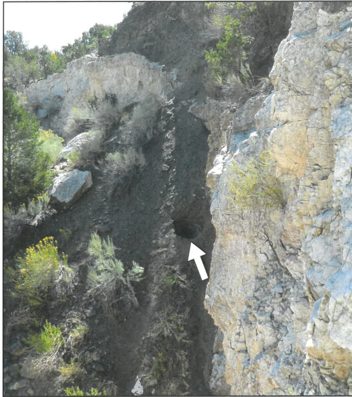
1 PHOTO OF SUB-2 LOCATION EXISTING CONDITIONS - LOOKING SOUTHEAST
