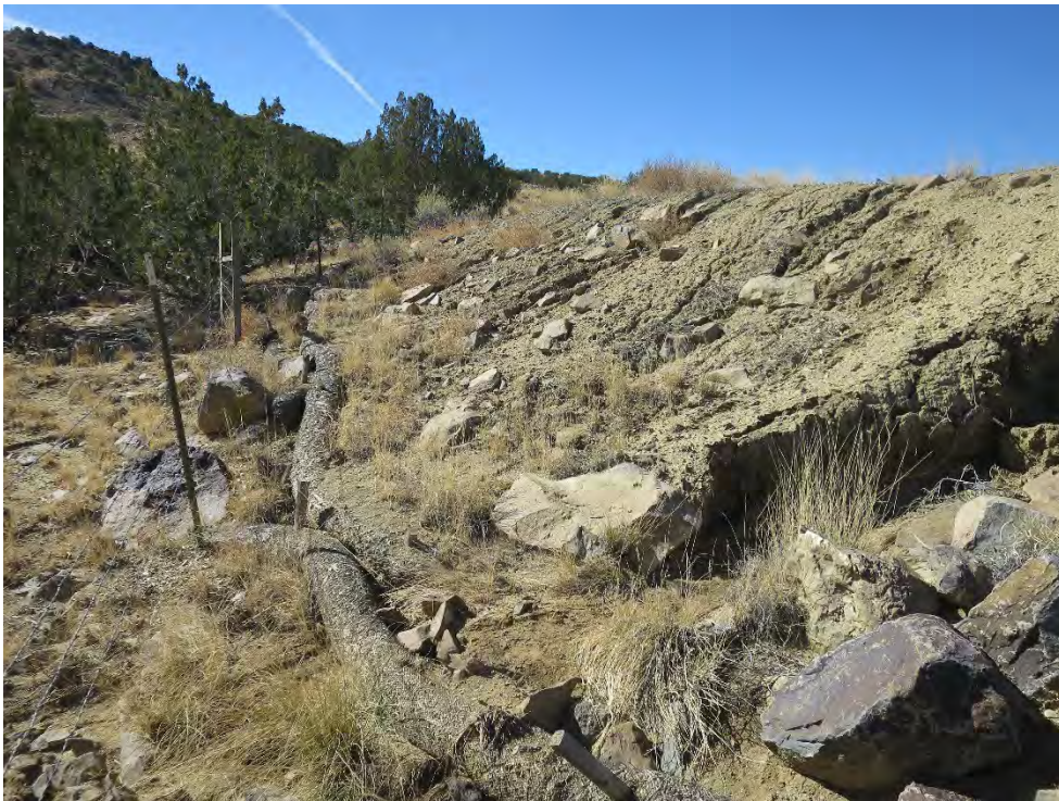
Photograph 22 - (VS-10 Photo Area D, looking east): Toe of slope in which a 3' deep channel has formed near the southeast fence line.
