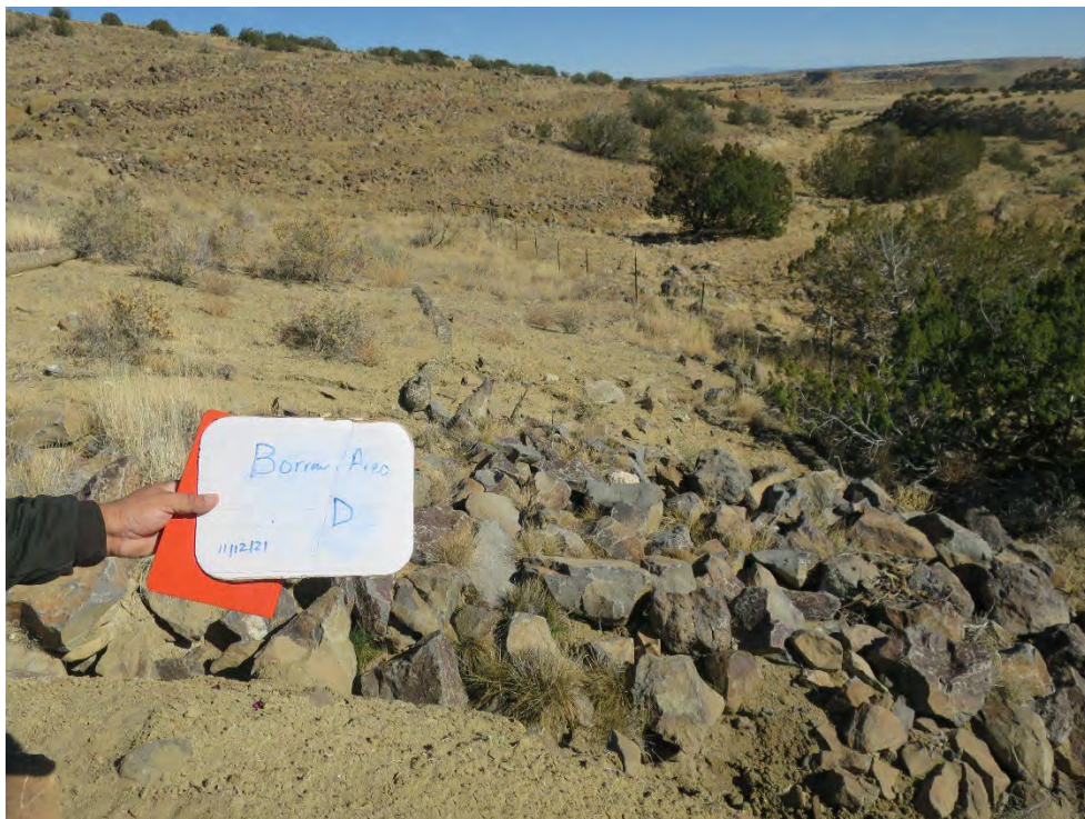
Photograph 20 - (VS-10 Photo Area D, looking east): Undercut and rilling along edge of existing rock armor.
