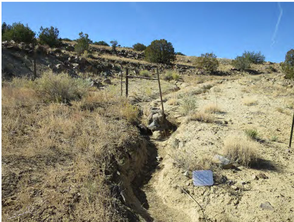
Photograph 37 - (VS-12 Photo Area D, looking west): Hay bales placed at VS-12 fence line. Note channel developing upstream near roadway and entering fence line, along the northwest side of VS-12.
