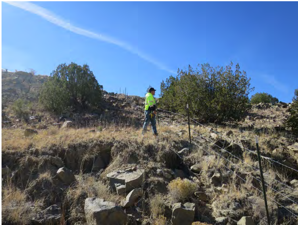
Photograph 39 - (VS-12 Photo Area F, looking southwest): Rilling present at the toe of hill at base of rock armoring.
