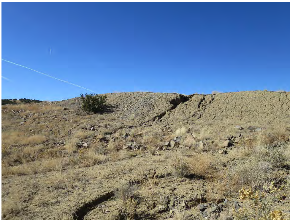
Photograph 26 - (Borrow Area/VS-10 Photo Area F, looking east): Erosion along steep slope between VS-10 and Borrow Area. Channel is about 5' to 7' wide and 5' deep near crest of the hill.
