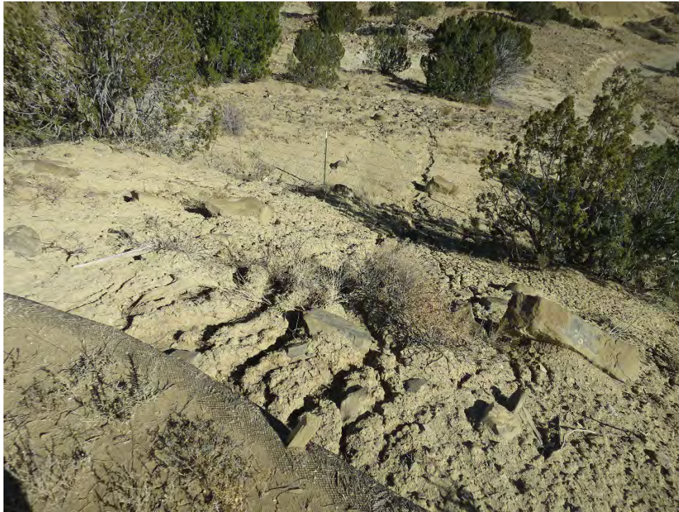
Photograph 34 - (VS-12 Photo Area B, looking northeast): Looking downhill from wood chip wattles. Wattles have provided some erosion protection. Rilling present on steeper downhill slope.
