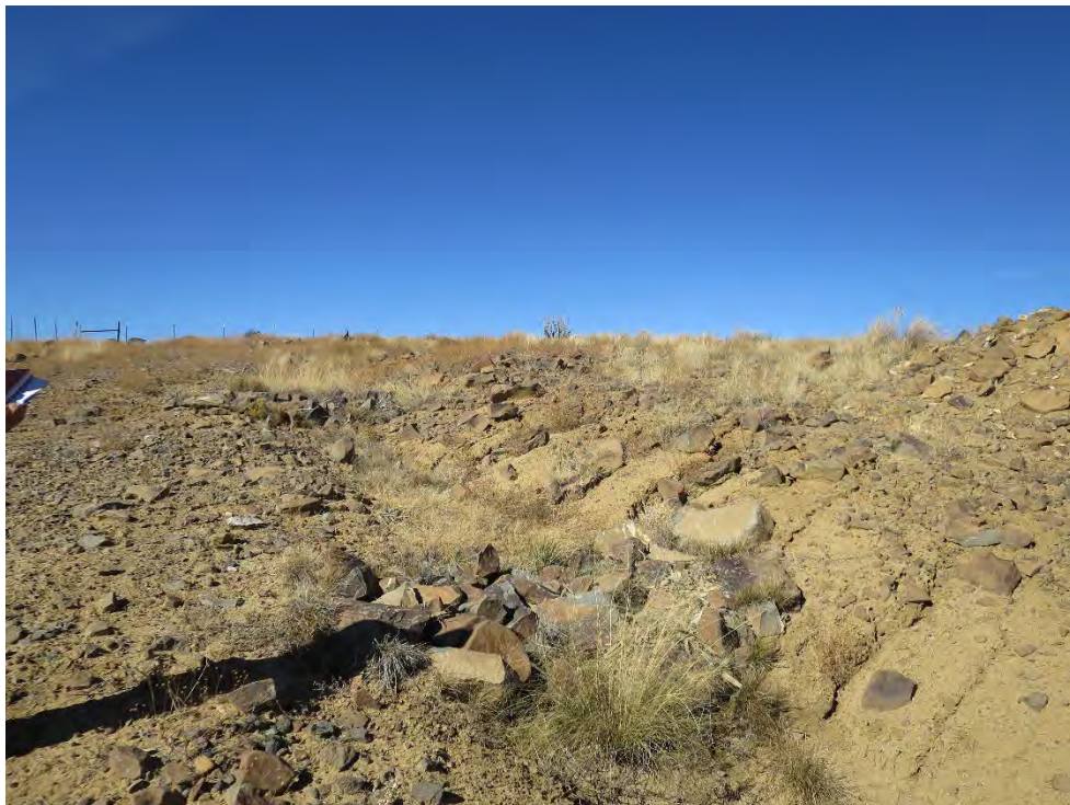
Photograph 18 - (VS-10 Photo Area B, looking west): Series of small rock check dams, with interrill-rill formation. The rill severity decreases as the slope flattens.
