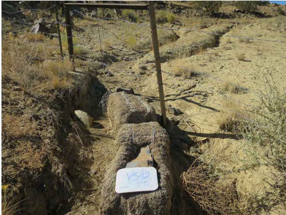
Photograph 38 - (VS-12 Photo Area D, looking west): Close-up of hay bales placed at VS-12 fence line ( 2014) to slow erosion.
