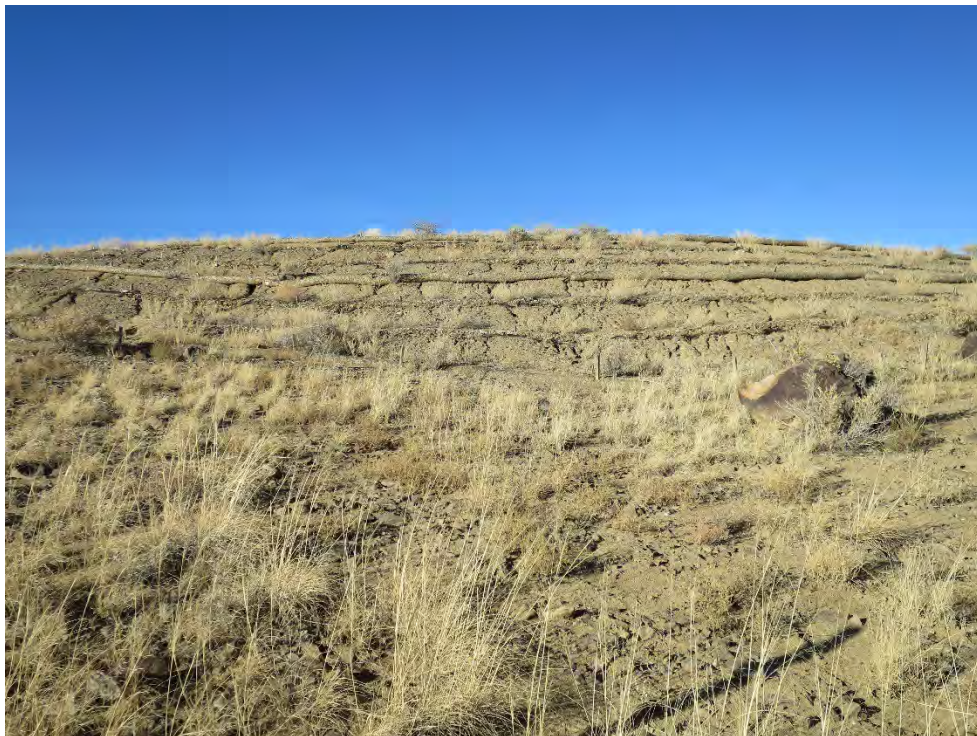
Photograph 41 - (Stockpile Photo Area B, looking north): Interrilling and rilling on all sides (south, east, and west) of the Stockpile hill despite wattles.
