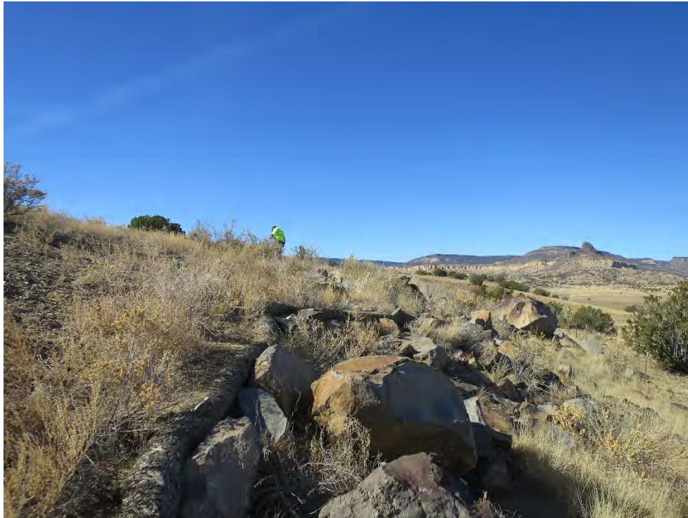
Photograph 3 - (VS-3 Photo Area B, looking north): Wood chip wattles and boulders used to control erosion within VS-3 fence line.
