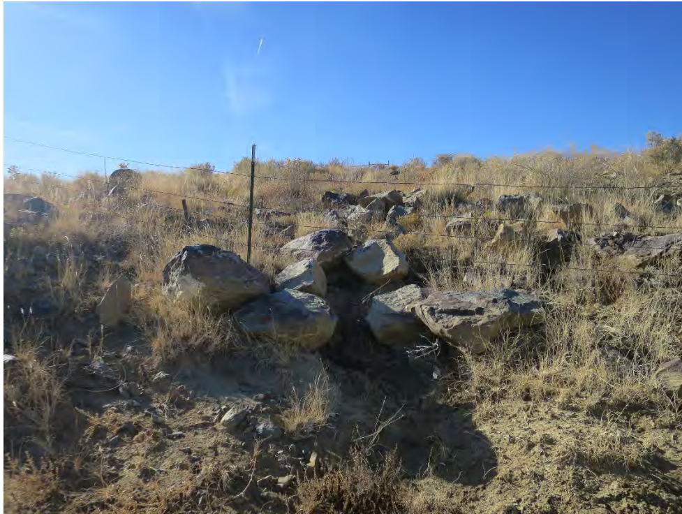
Photograph 9 - (VS-5 Photo Area C, looking west): Moderate undercutting starting within armored zone within the fenced area.
