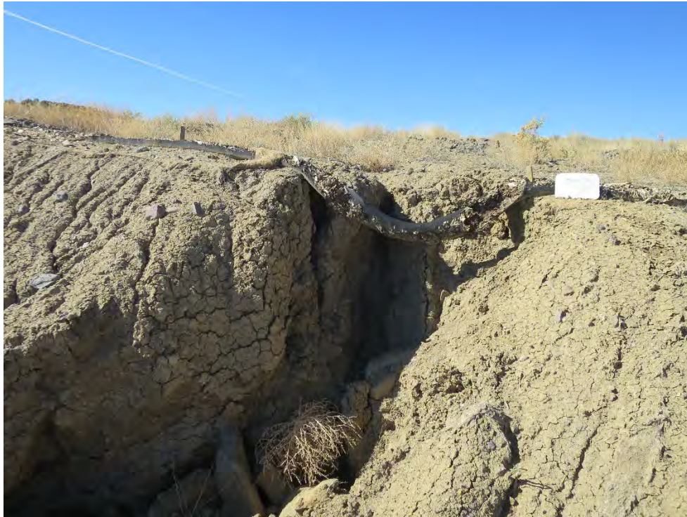
Photograph 27 - (Borrow Area/VS-10, looking northwest): Closeup of deep erosional channel at the crest of the hill between the Borrow Area and VS-10.
