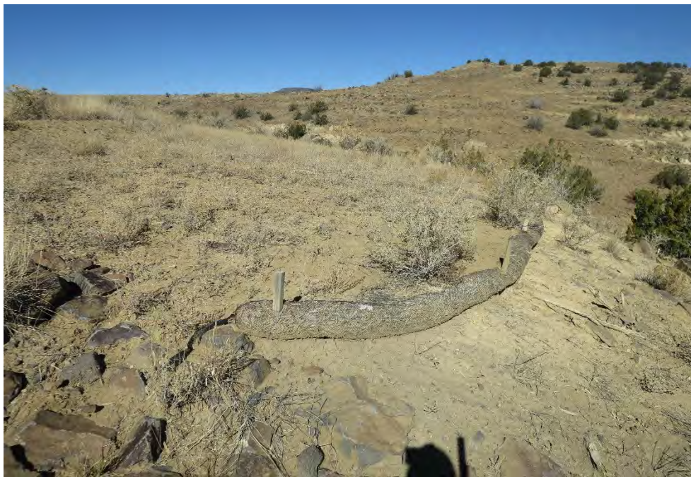
Photograph 33 - (VS-12 Photo Area B, looking northwest): Wood chip wattles providing erosion protection. Interrilling present below wattles.
