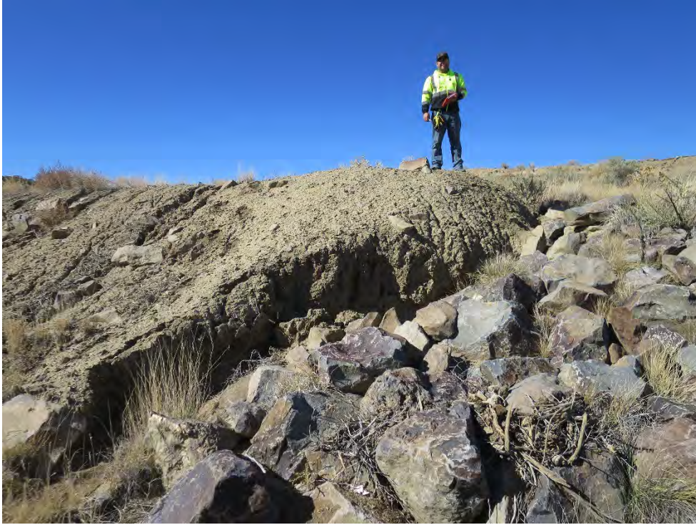
Photograph 21 - (VS-10 Photo Area D, looking northwest): Gully erosion along edge of existing rock armor, forming channels into slope.
