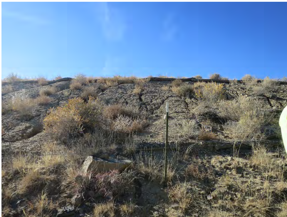
Photograph 8 - (VS-5 Photo Area B, looking west): Interrill and gully formation on slope below wattles within the fence line.
