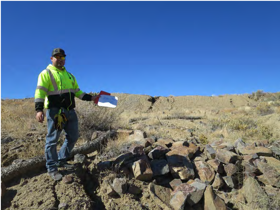
Photograph 24 - (Borrow Area/VS-10 Photo Area F, looking northeast): Significant gully erosion, creating channels along steeper slopes.
