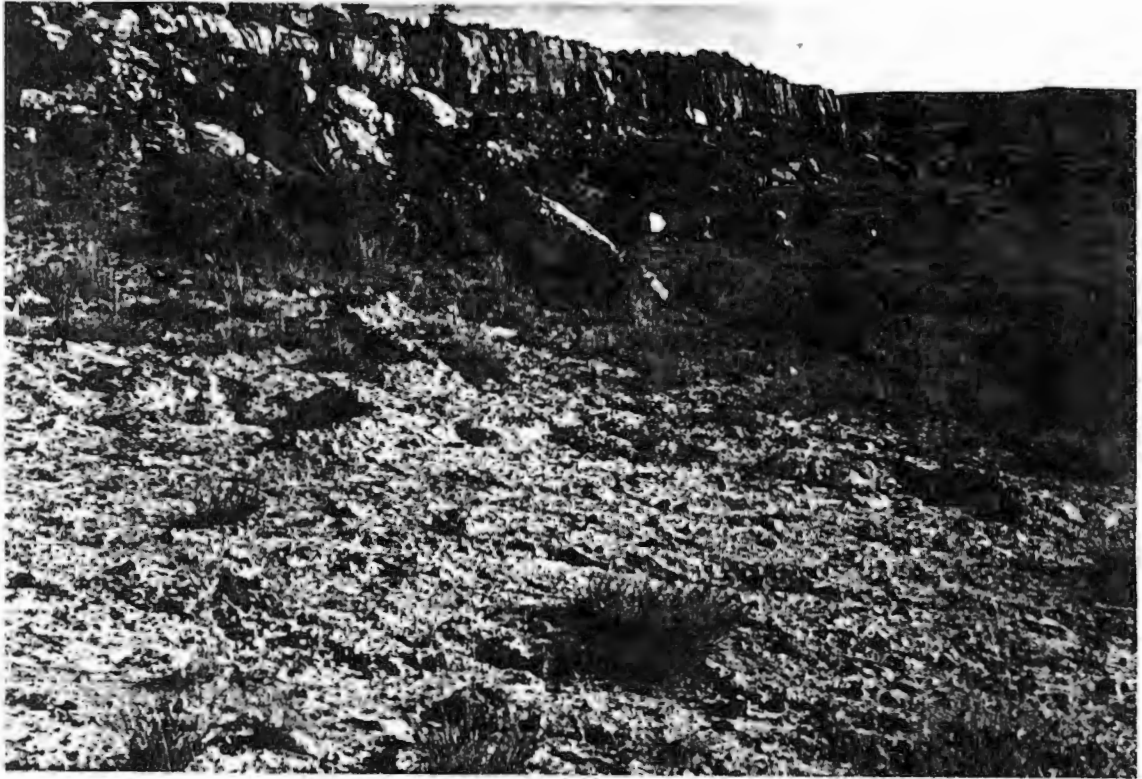
PHOTO 7 - East slope of Doris waste pile, showing low earth berms along contours to control runoff.
