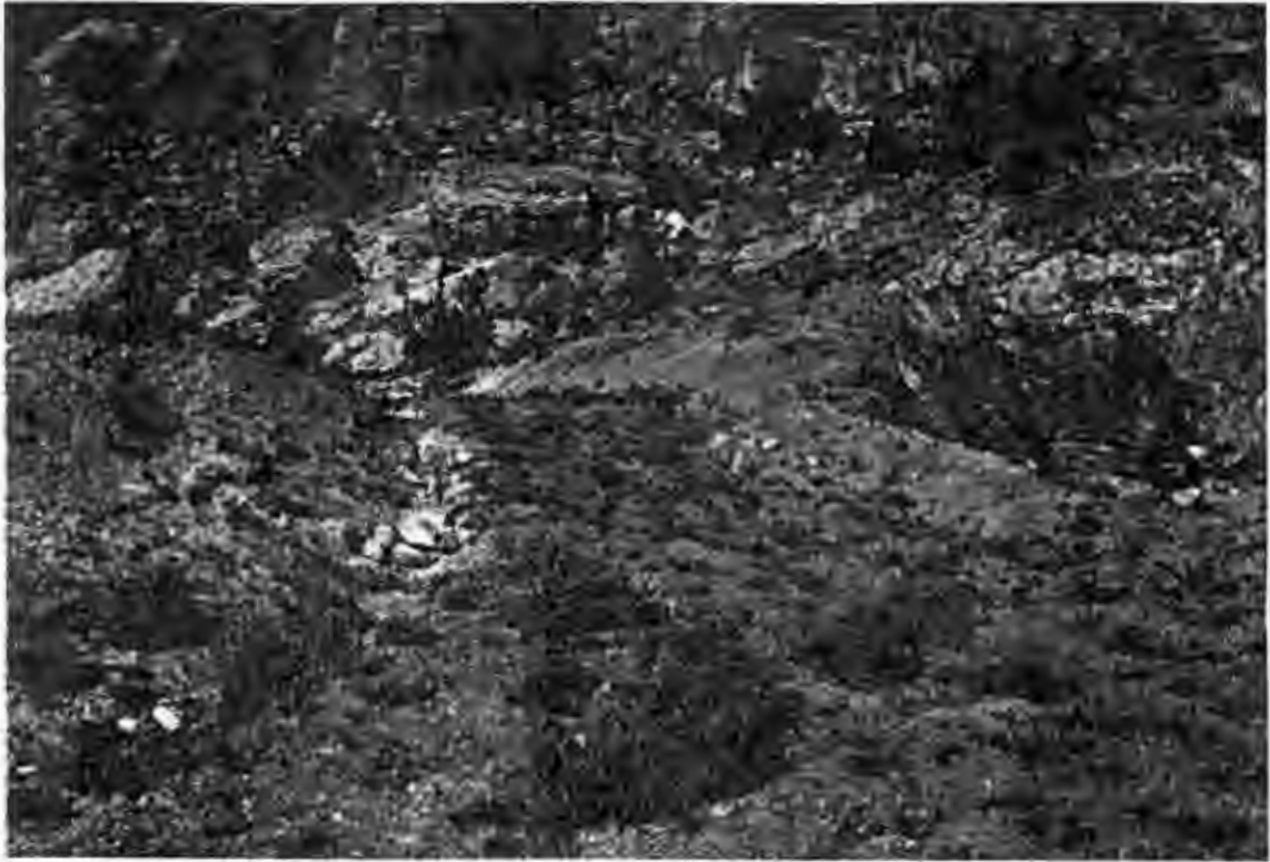
PHOTO 5 - North end of main decline access road showing rock check dams along ditches each side of road.
